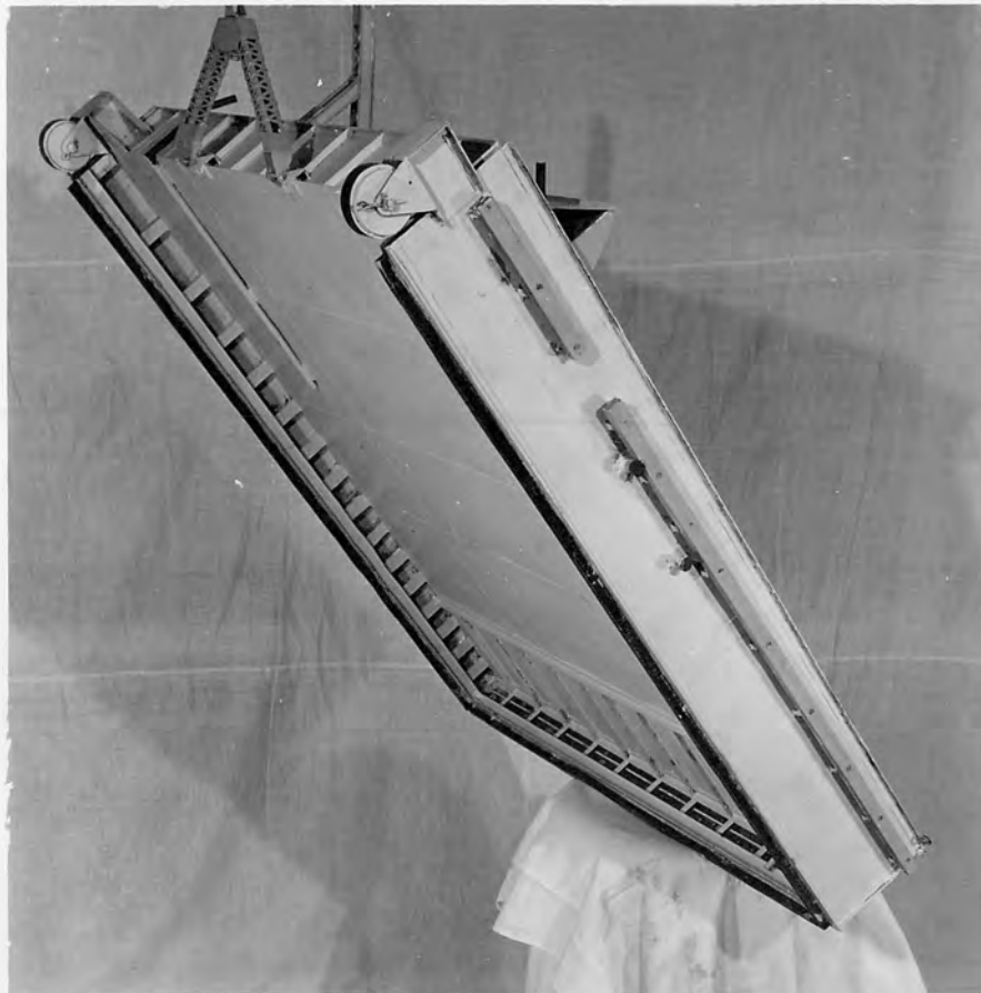
B. Caisson tilted to show working space on under side.
