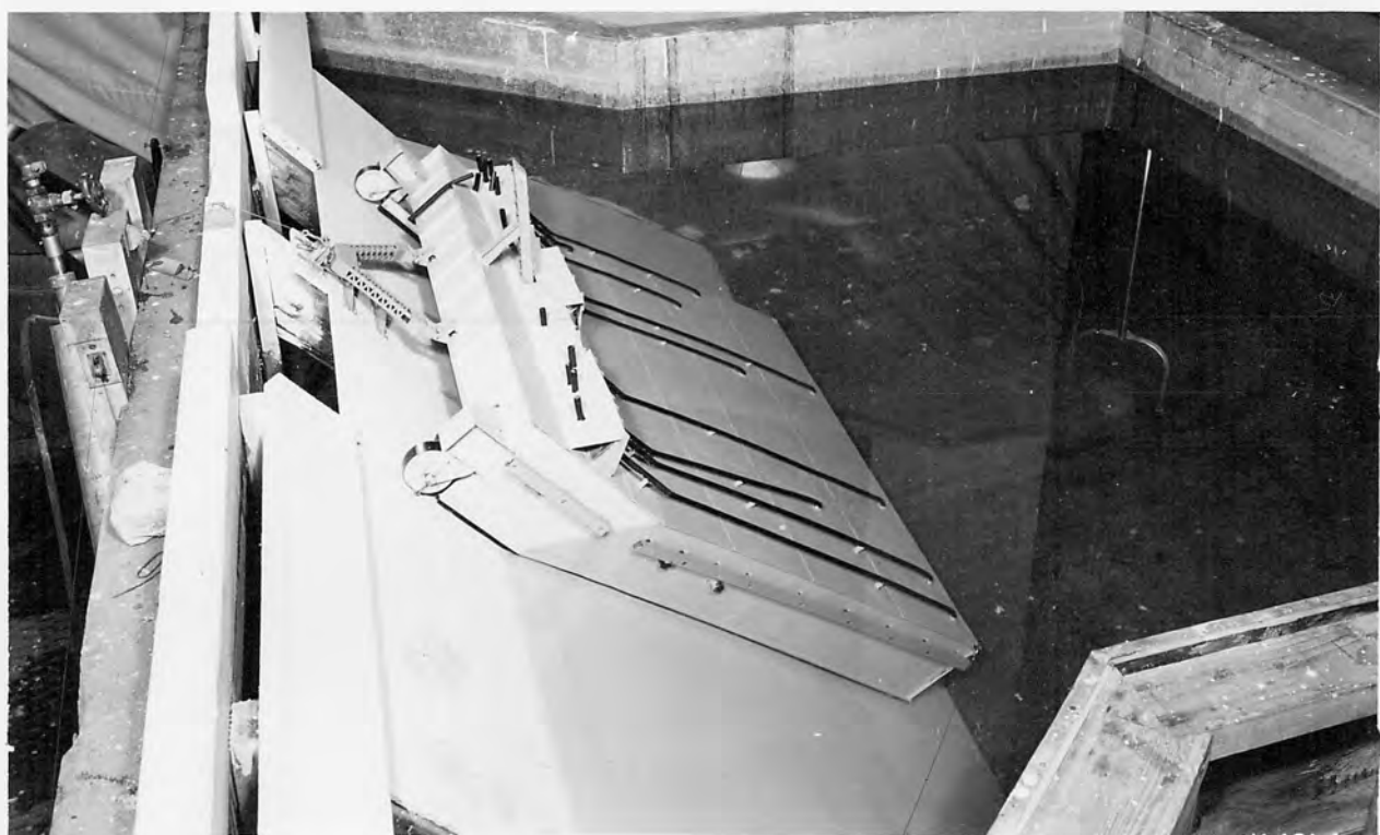
B. Caisson sealed preparatory to unwatering work chamber.
