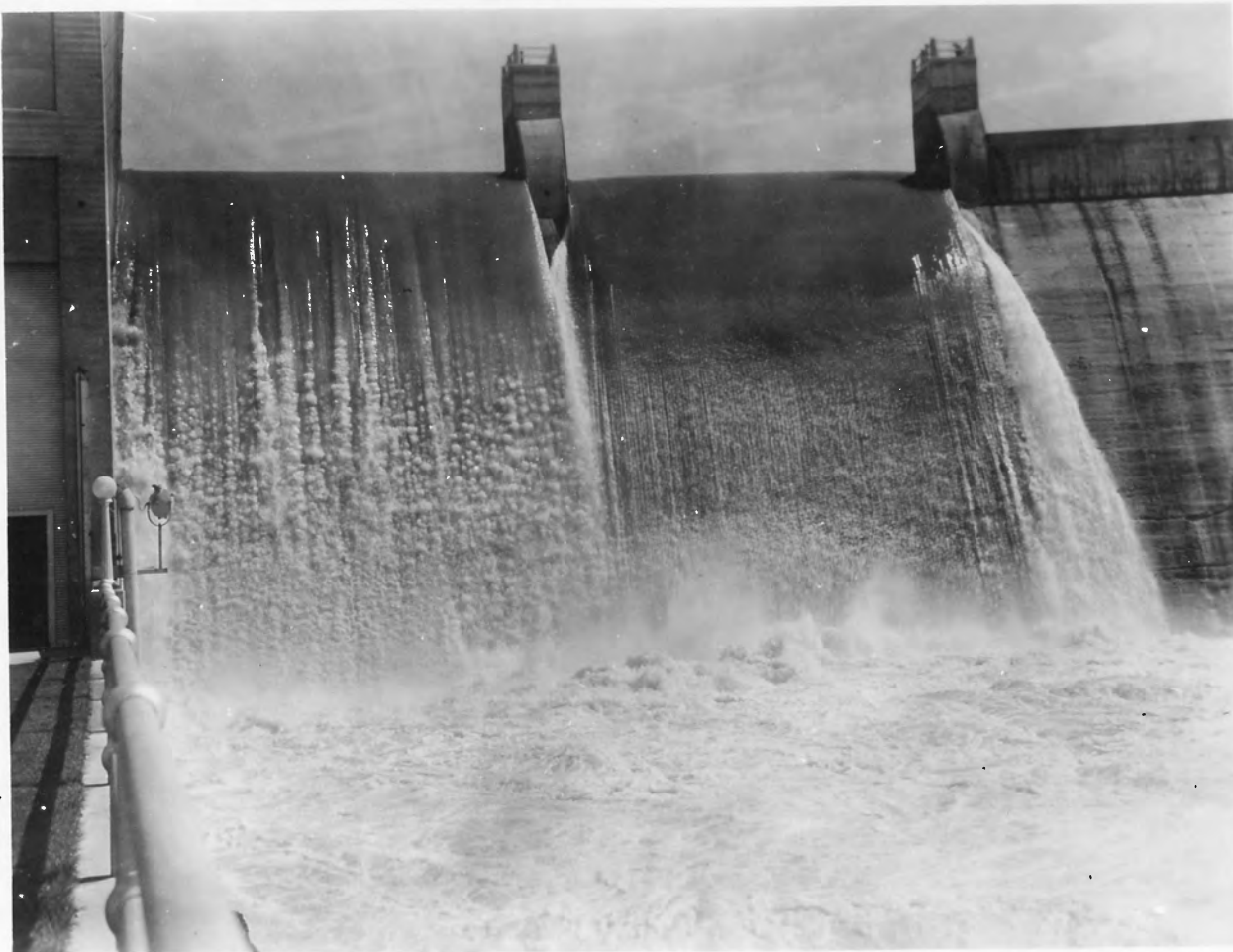
SPILLWAY CONTROLLED BY THREE 64 BY 14.5-FOOT DRUMGATES CENTER GATE COMPLETELY LOWERED - HEAD 6.5 FEET GATE NO. 3 RAISED 2 FEET DISCHARGE TWO GATES, APPROXIMATELY 6,000 SECOND FEET TOTAL DROP, HEADWATER TO TAILWATER 81 FEET BLACK CANYON DAM
