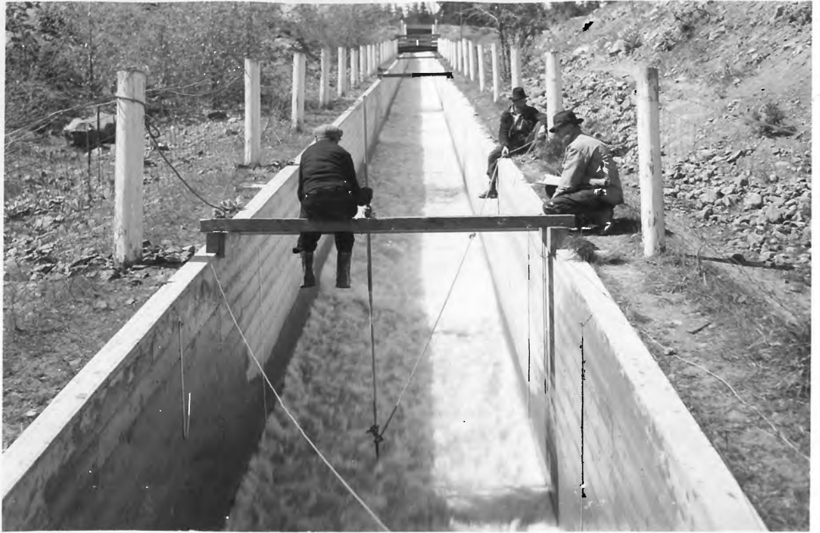
A. POINT GAGE USED FOR OBTAINING DEPTH OF FLOW.
