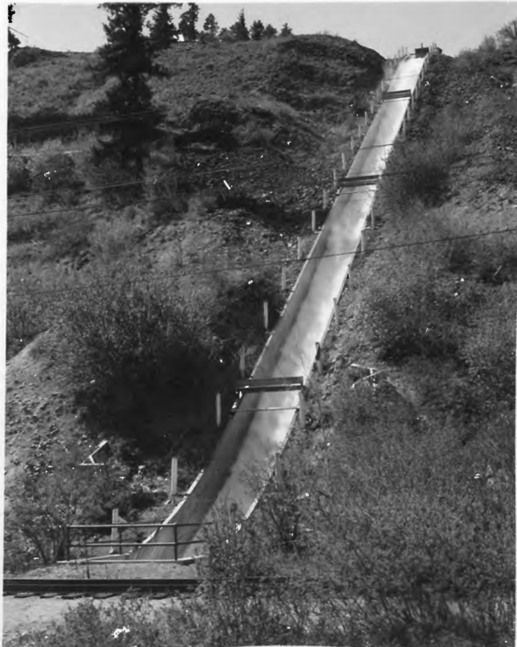
B. FLOW CONDITIONS ON 33^{\circ} - 10' SLOPE. DISCHARGE 922 SECOND-FEET
