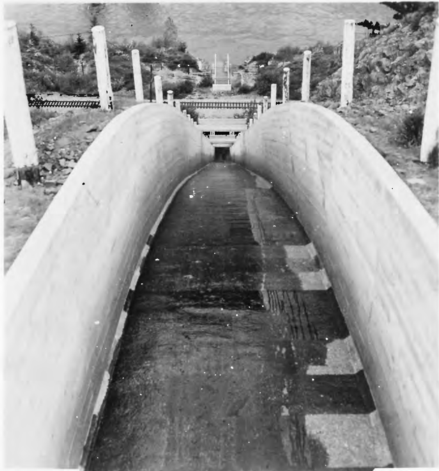
B. LOWER SECTION OF WASTEWAY - LOOKING DOWNSTREAM
