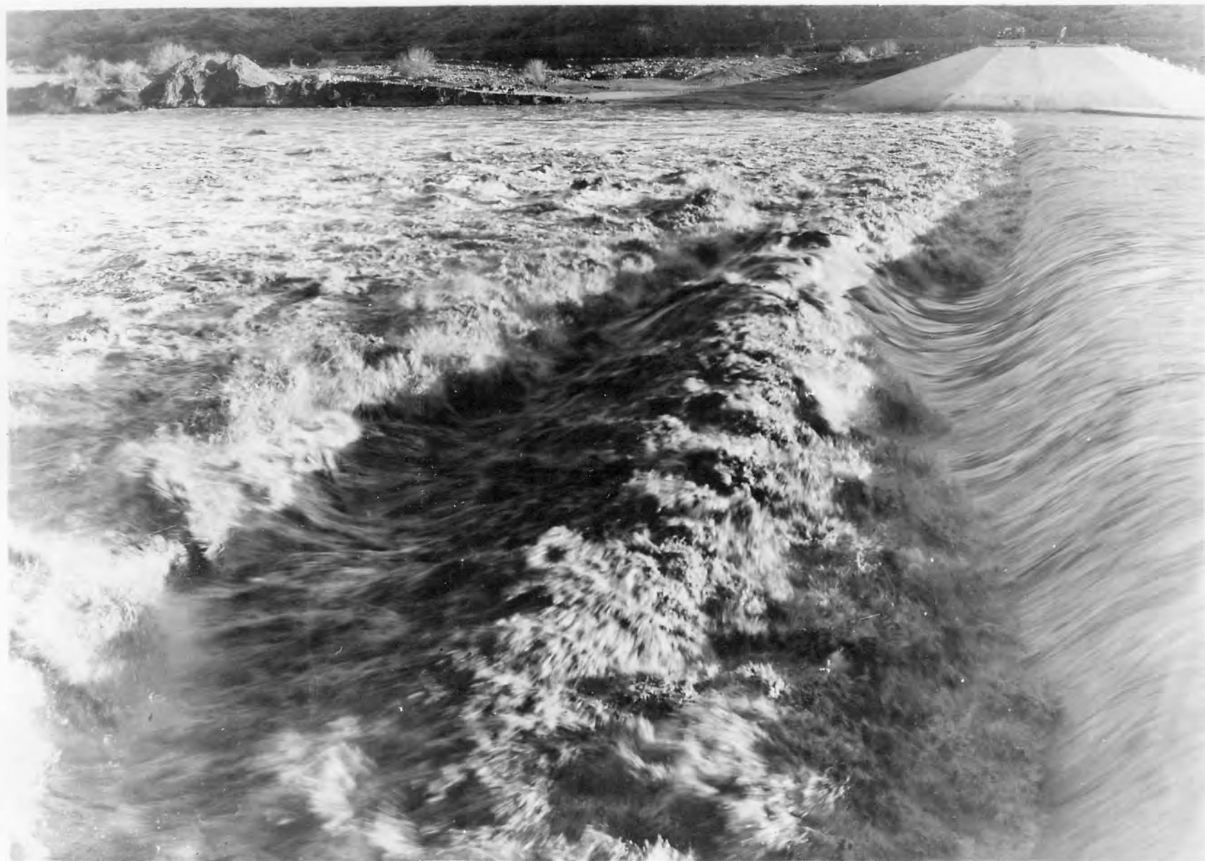
VIEW OF PROTOTYPE FROM LEFT BANK SHOWING CONCENTRATION OF FLOW NEAR LEFT END OF SPILLWAY FOR A DISCHARGE OF 38,000 SECOND-FOOT.
