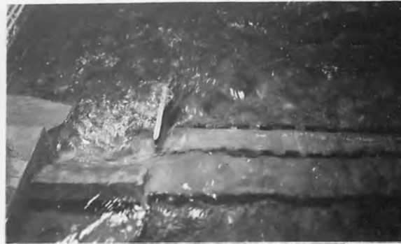
B. Discharge 150,000 second-feet
