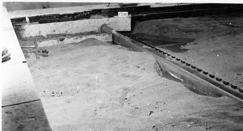
PITS ADJACENT TO UPSTREAM FACE OF DAM NEAR THE LEFT END.
