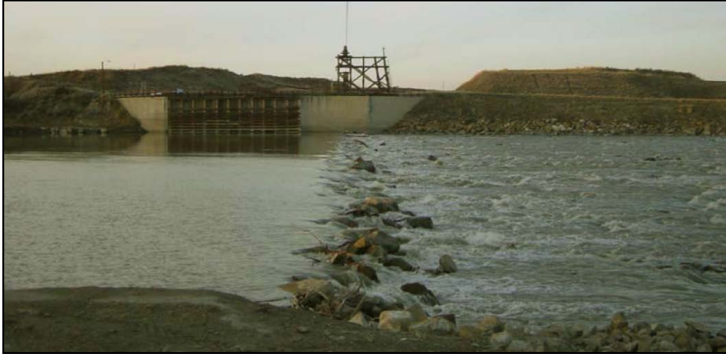
Figure 2. Lower Yellowstone Diversion Dam today with large rock dumped along the dam crest that has migrated downstream over the years preventing fish passage.
