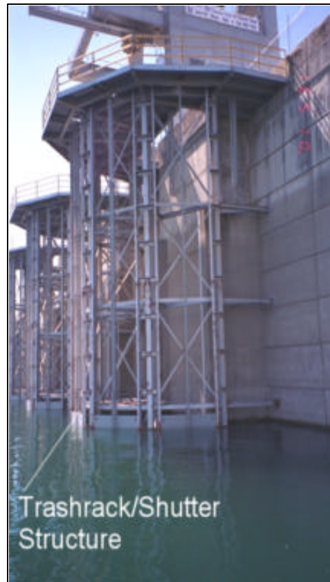
Figure 2. Photograph of Folsom shutter guides and panels.
