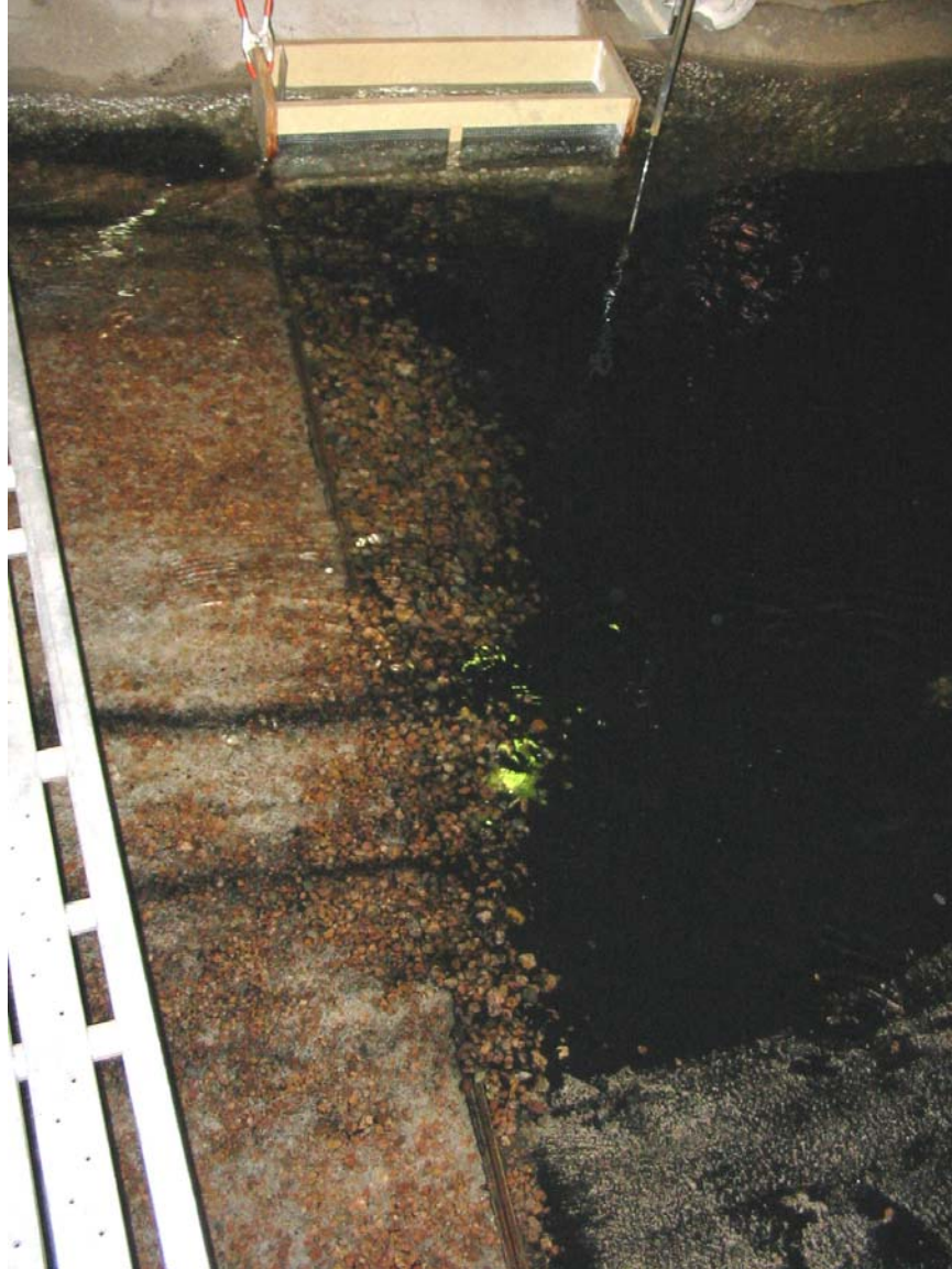
Photograph 13.—View of bed material moving across the dam crest near the left bank during a flow of 6,500 ft 3 /s.
