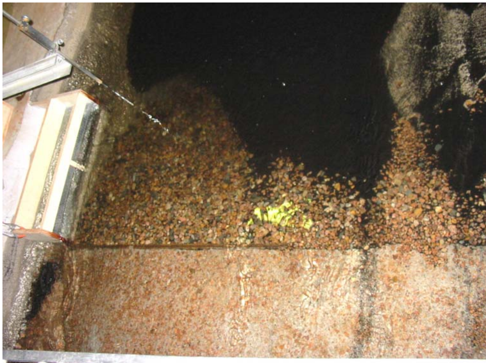
Photograph 18.—View looking down on the dam crest following the 10,000 ft 3 /s hydrograph test. Flow shown is 2,000 ft 3 /s.
