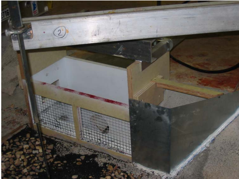
Photograph 23.—View of the upstream guide wall modification to the intake structure.
