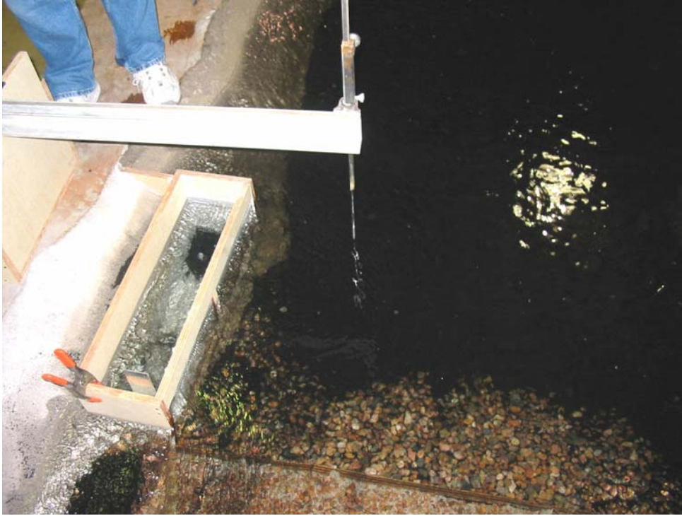
Photograph 14.—View of bed sediment moving across dam crest and down the low-flow channel during peak flow conditions.
