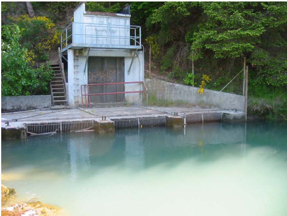
Photograph 2.—View of existing Elwya surface-water intake structure.
