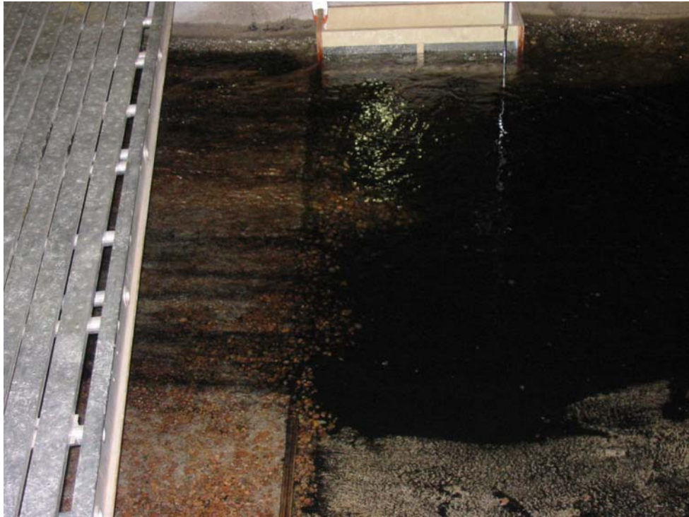
Photograph 16.—View of 10,000 ft 3 /s river flow showing transport of bed sediments across the dam crest.
