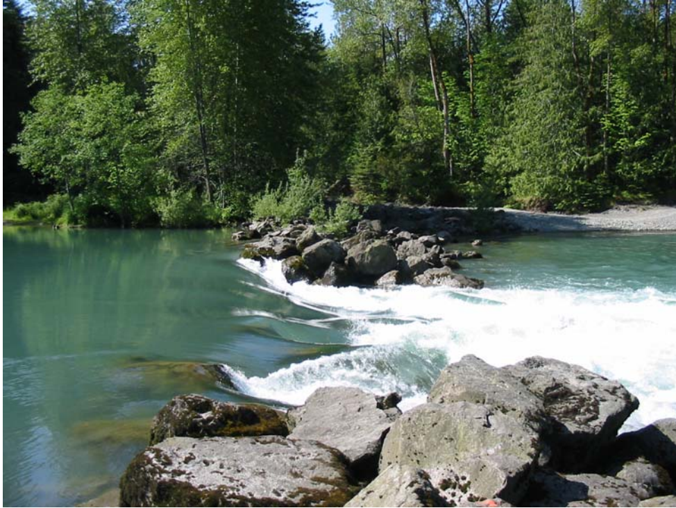
Photograph 1.—View looking from the right bank across the existing Elwya surface-water intake diversion dam.
