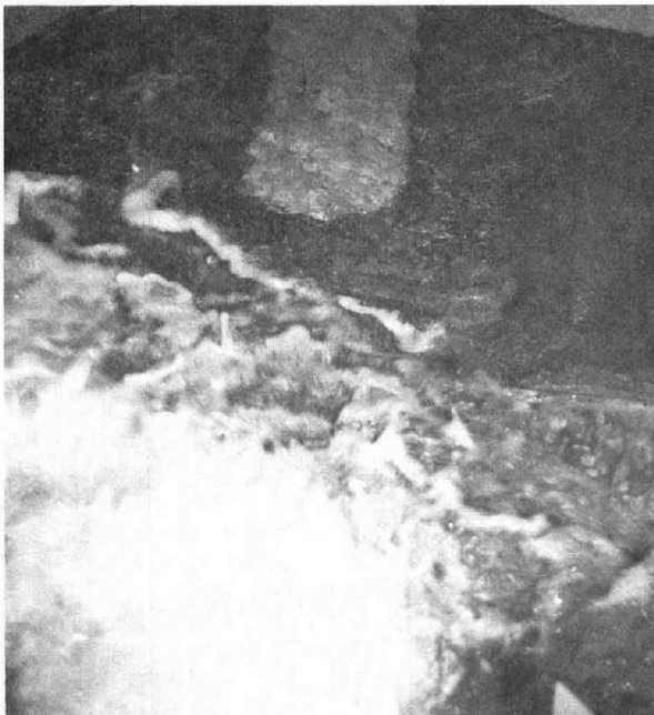
c. Downstream channel during sweepout. Photo P801-D-79462
