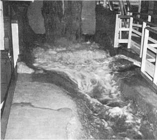
FIGURE 20.—View showing flow in unmodified powerplant tailrace with all gates fully open (approximate discharges: spillway Q=40,000 cubic feet per second, outlet works Q=1,500 cubic feet per second, powerplant Q=5,200 cubic feet per second).
