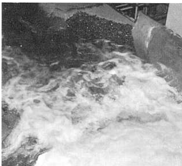
FIGURE 26.—Flow conditions downstream from the weir after excavation of talus slope on the right bank (approximate discharges: spillway Q=34,400 cubic feet per second, outlet works Q=1,500 cubic feet per second, and powerplant Q=5,200 cubic feet per second).
