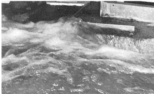
FIGURE 24.—Test of floodwall protection around visitors' center (approximate discharges: spillway Q=32,900 cubic feet per second, outlet works Q=1,500 cubic feet per second and powerplant Q=5,200 cubic feet per second).
