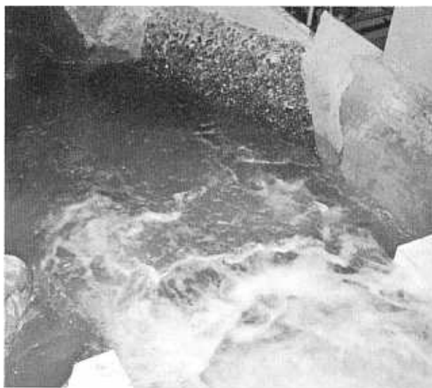
FIGURE 25.—Flow conditions downstream from the weir after excavation of talus slope on the right bank (approximate discharges: spillway Q=17,200 cubic feet per second, outlet works Q=1,500 cubic feet per second, and powerplant Q=5,200 cubic feet per second).
