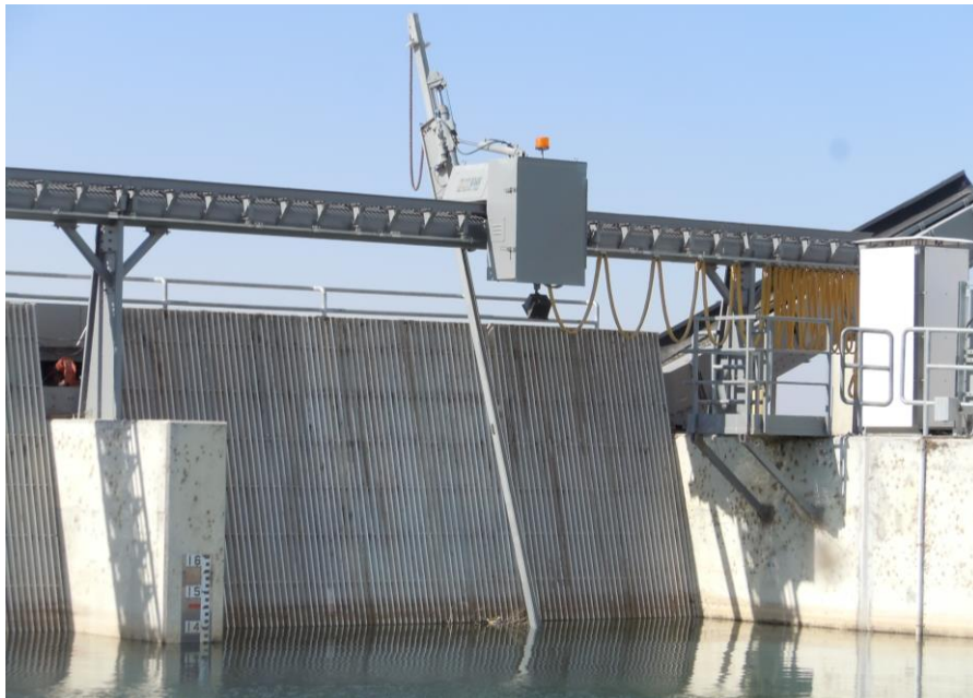
Figure 12.2.1.1-1. End bearing trashracks located within a canal. Trashracks were provided with automated trash rake and conveyor debris removal system.
