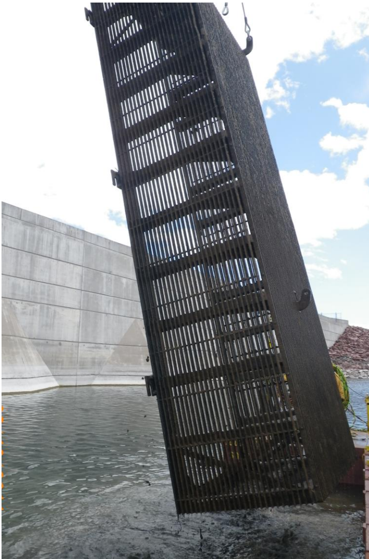
Figure 12.2.1.3-1. Three-sided integral trashracks being reinstalled over dam outlet works.
