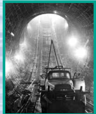
1956 work on Palisades Dam
