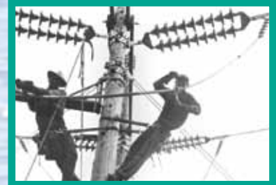
Early transmission line work
