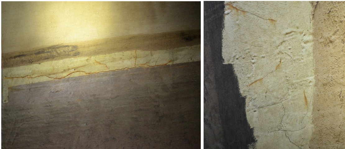
Photo 23. Cracked coating
