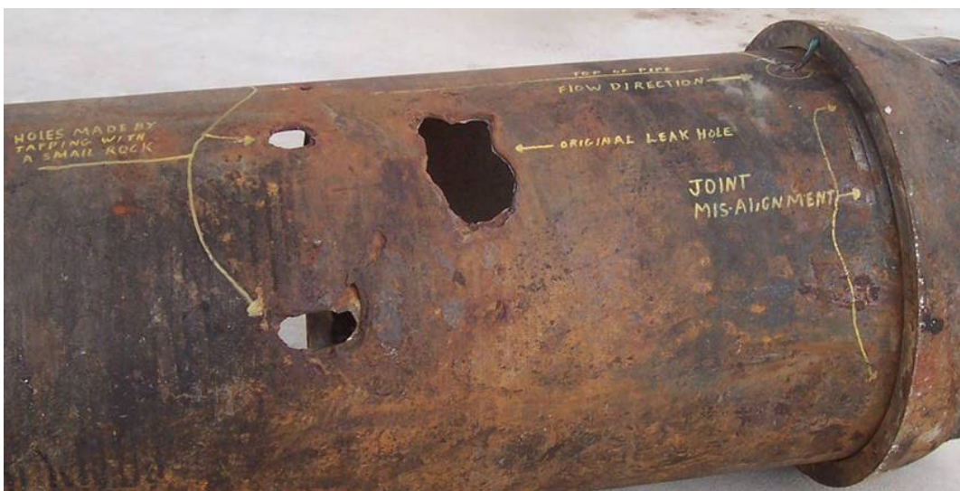
Photo 6. Failed pipe demonstrating selective leaching.
