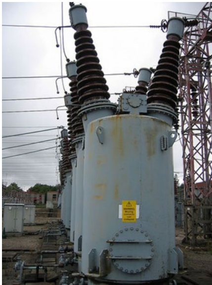
Figure 7-1. Oil circuit breaker
