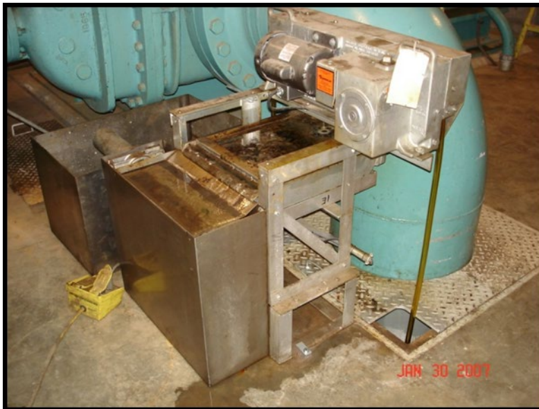
Photograph 1.—Plant sump oil skimmer assembly.
