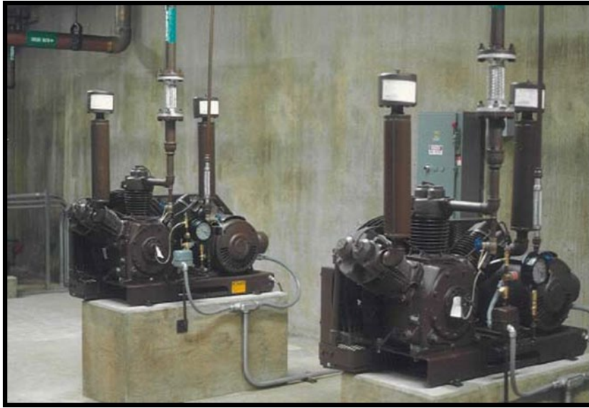
Photograph 13.—Reciprocating type air compressors.
