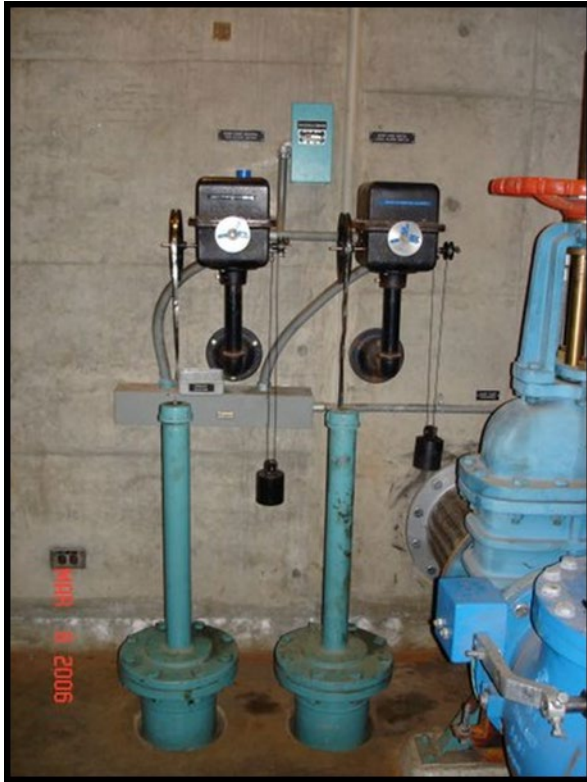
Photograph 3.—Float operated sump-water-level monitoring and indicating systems.
