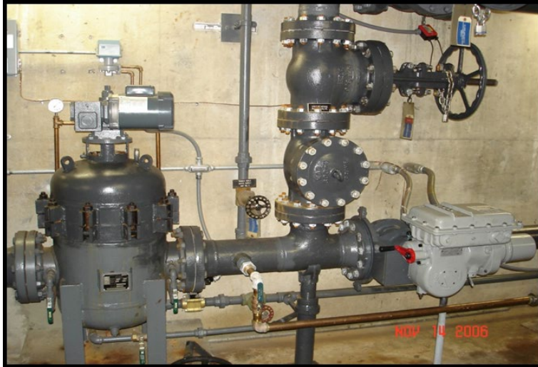
Photograph 5.—Automatic, self-cleaning, moto-operated strainer and associated piping components.
