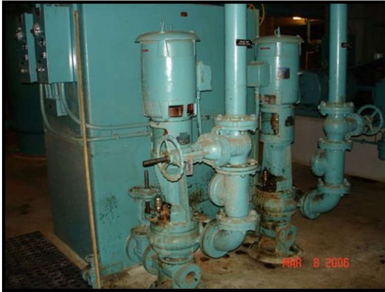
Photograph 9.—Sewage pumping units and collection reservoir tank.
