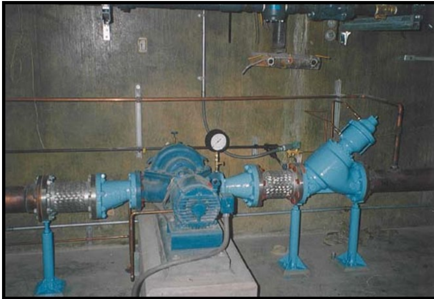
Photograph 4.—Unit cooling water pump assembly.
