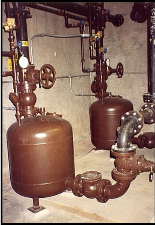
Photograph 8.—Pneumatic duplex sewage ejectors.
