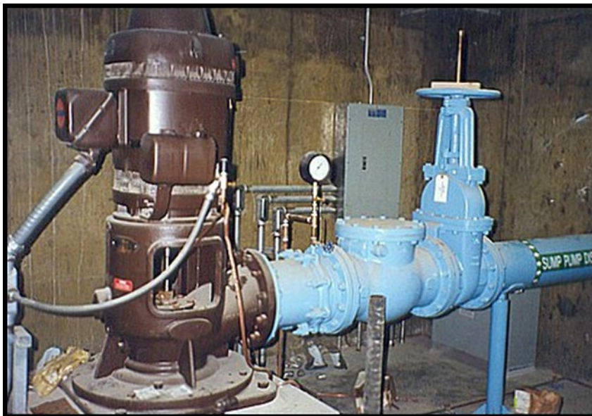
Photograph 2.—Sump pumping unit discharge assembly.
