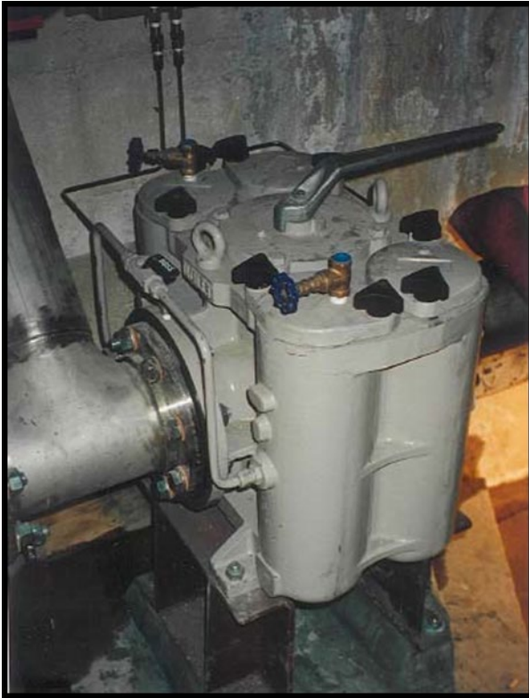
Photograph 6.—Manual basket duplex strainer.
