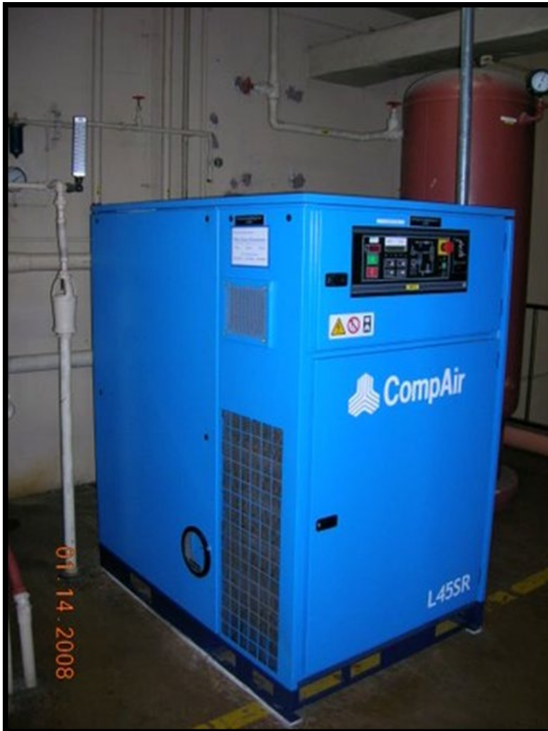
Photograph 14.—Rotary screw type air compressor.
