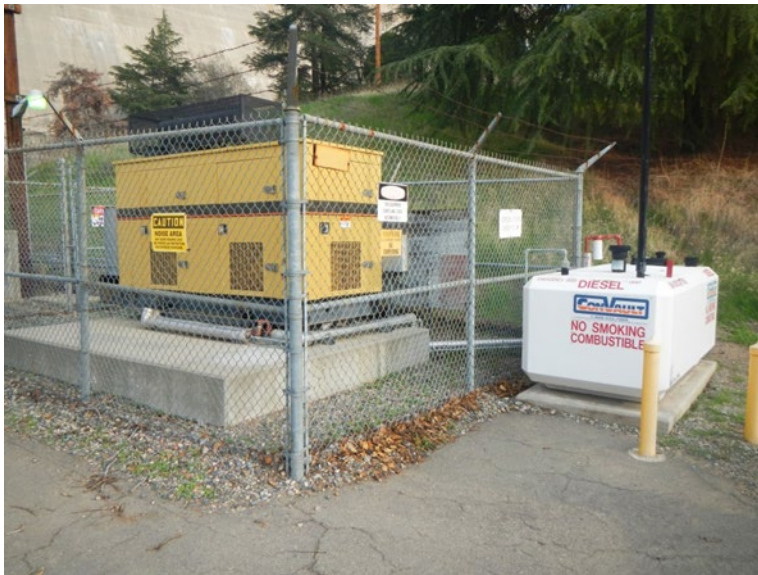
Photograph 15.—Engine generator set and fuel supply tank.
