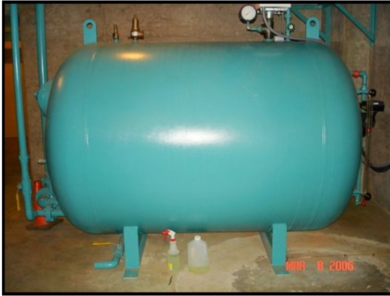
Photograph 7.—Service-water hydropneumatic tank.
