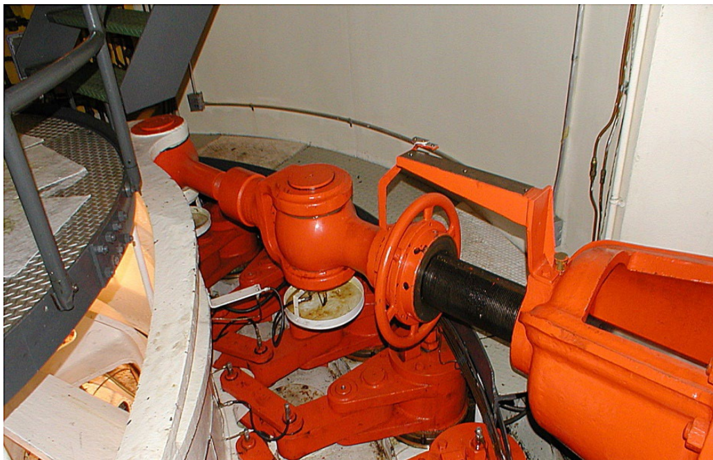
Photo 7.—Servomotor connecting rod.
