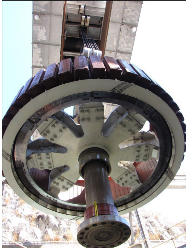
Photo 18.—Rotor assembly.
