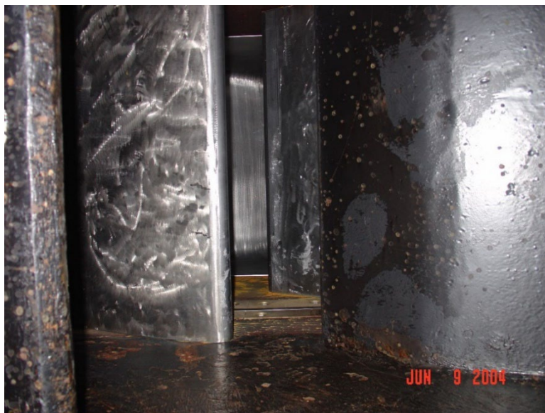
Photo 5.—Wicket gates and stay vanes.
