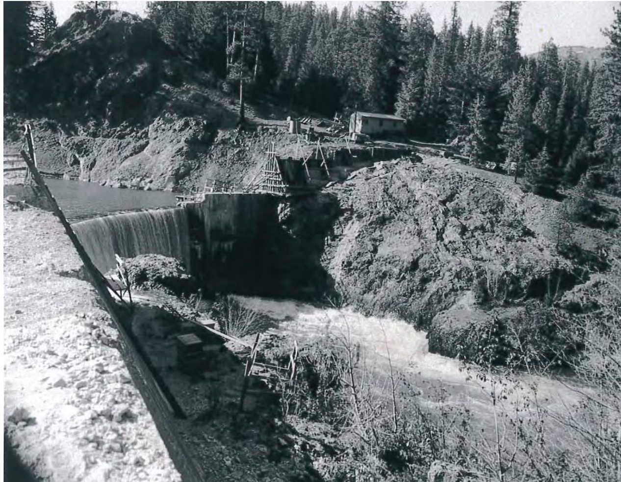
Clear Creek Dam repairs circa 1965
