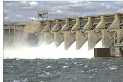
Ice Harbor Dam Tailrace, Lower Snake River (2023)
