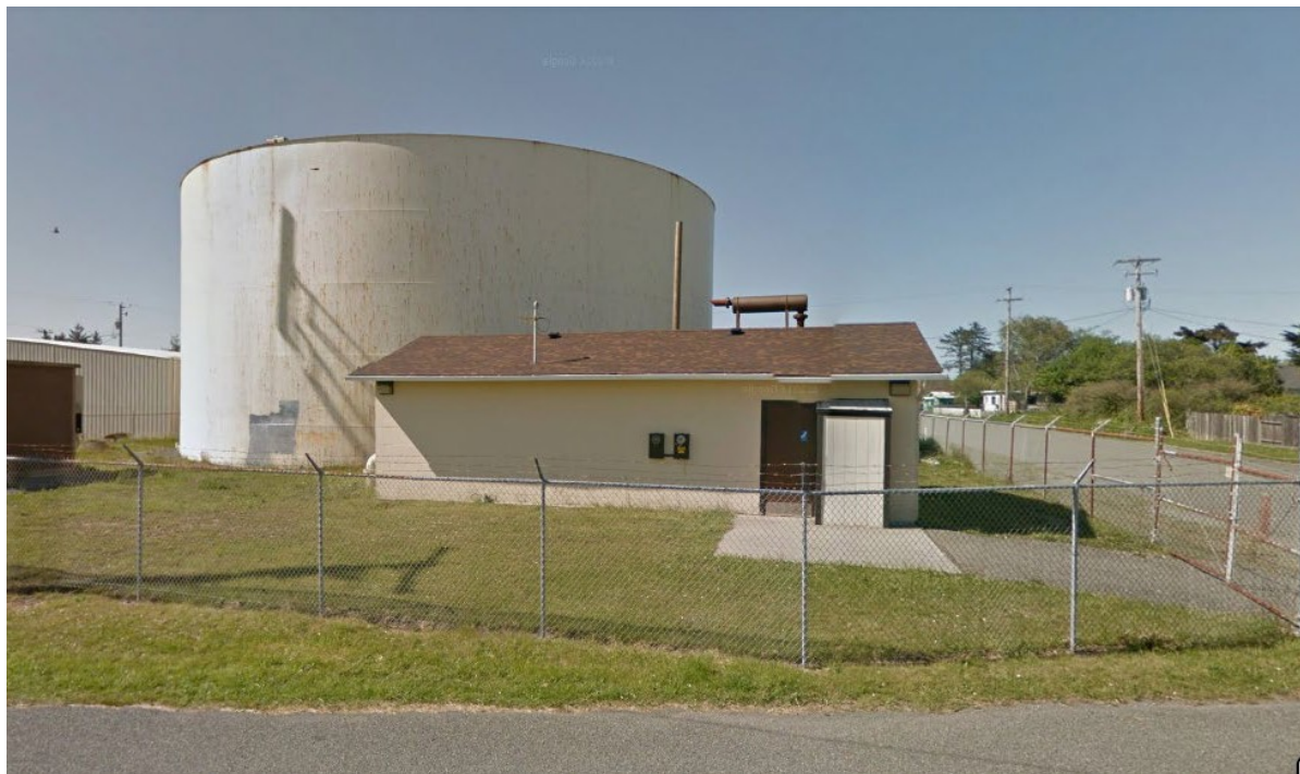
Figure 1- Amador Water Tank
