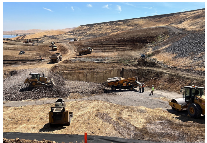
Construction is underway to improve the seismic reliability of B.F. Sisk Dam; it is Reclamation's largest project under the 1978 Dam Safety Act.
