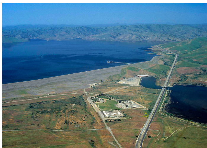
Raising B.F. Sisk Dam and expanding San Luis Reservoir will create an additional 130,000 acre-feet of needed water storage south-of-the-Delta—enough water supply for two million people, over one million acres of farmland, and 135,000 acres of Pacific Flyway wetlands.
