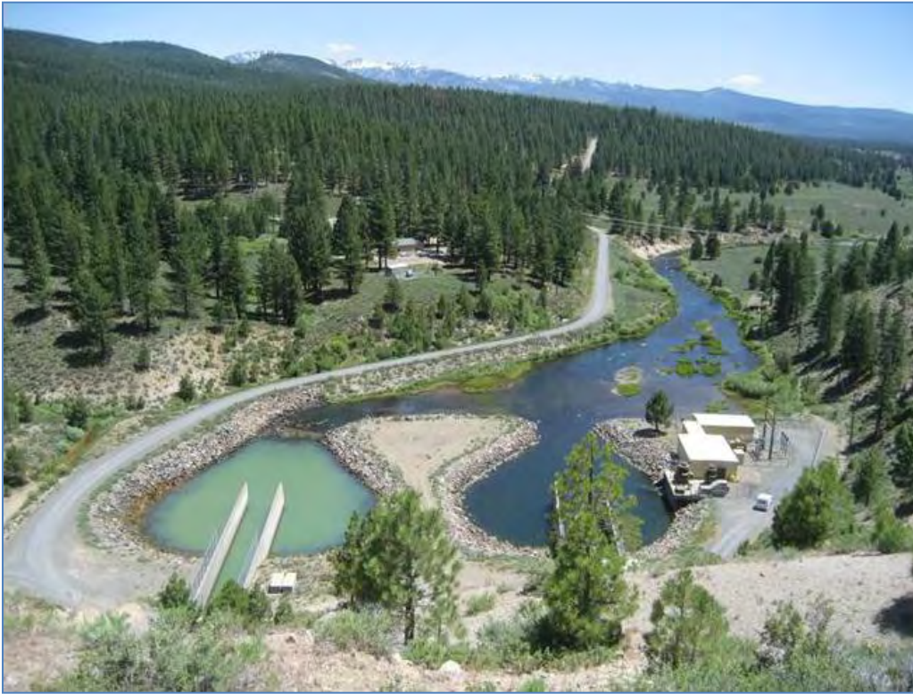
Figure 1-6.—Spillway, outlet works, and Stampede Powerplant located below Stampede Dam.
