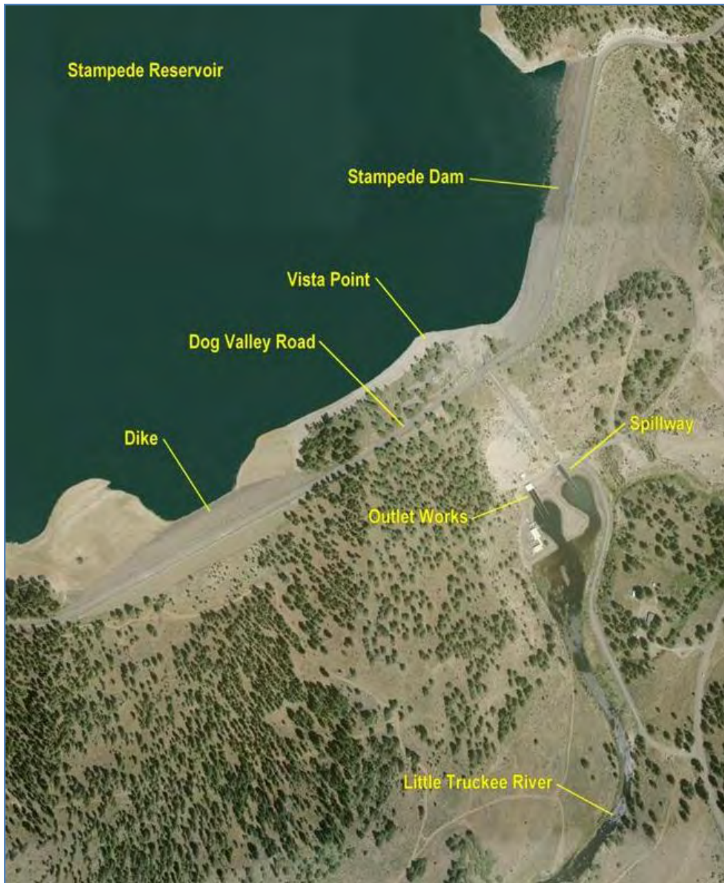
Figure 1-3.—Stampede Dam features.
