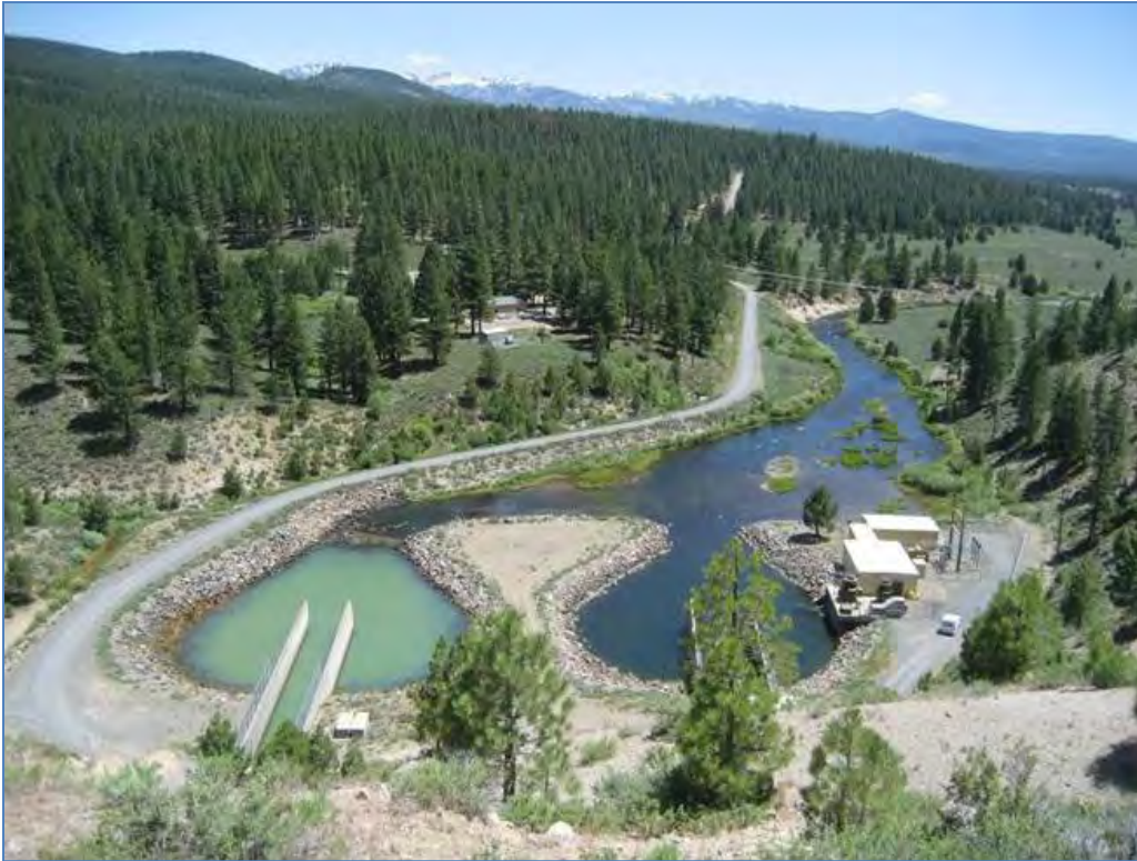
Figure 1-6.—Spillway, outlet works, and Stampede Powerplant located below Stampede Dam.
