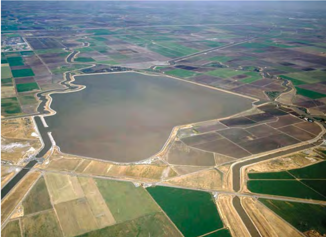
Clifton Court Forebay
