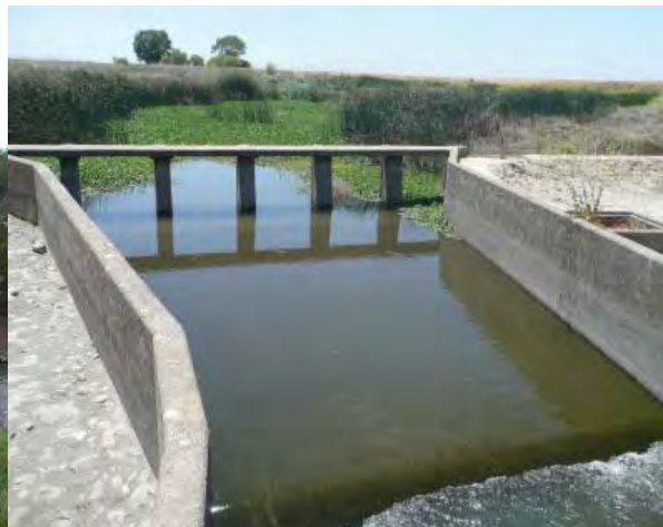
Sand Slough Control Structure
