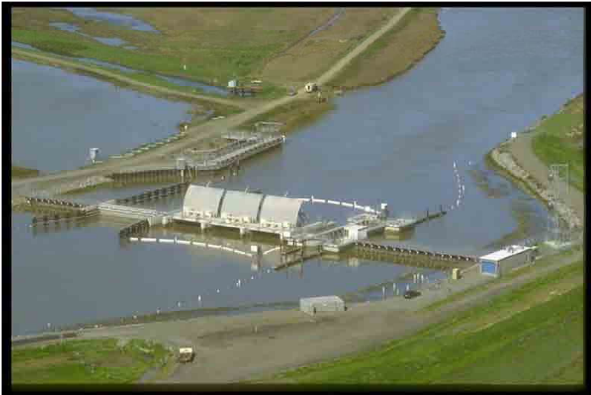
Figure 3-14 Aerial view of the Suisun Marsh Salinity Control Gates.
