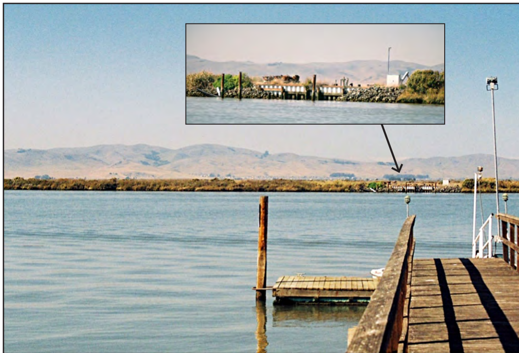
Photo 4. This photo depicts common infrastructure in the marsh including a pier and pylons, outfall structure, and riprap (inset). The building in the inset photo is the lower Joice Island Fish Screen Facility.
