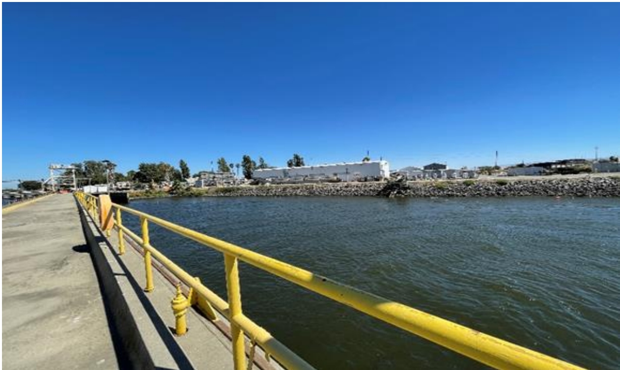
Figure A-12. Picture of Tracy Fish Collection Facility
