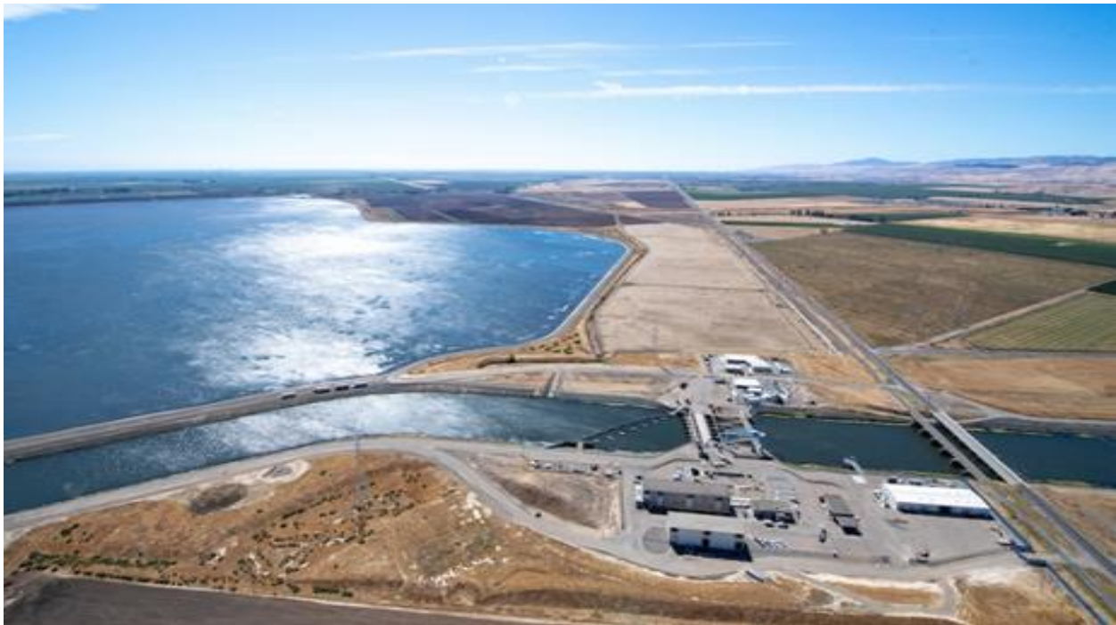
Figure A-40. Picture of Clifton Court Forebay and John E. Skinner Delta Fish Protective Facility
