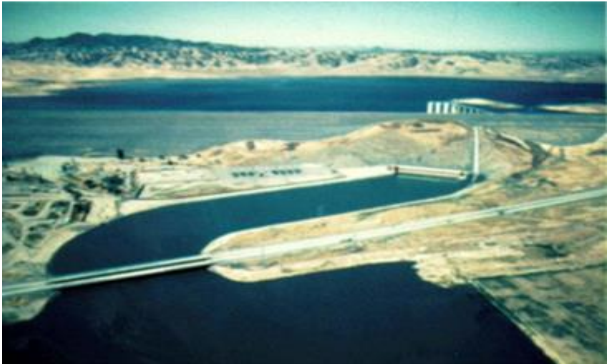
Figure A-36. Picture of William R. Gianelli Pumping-Generating Plant
