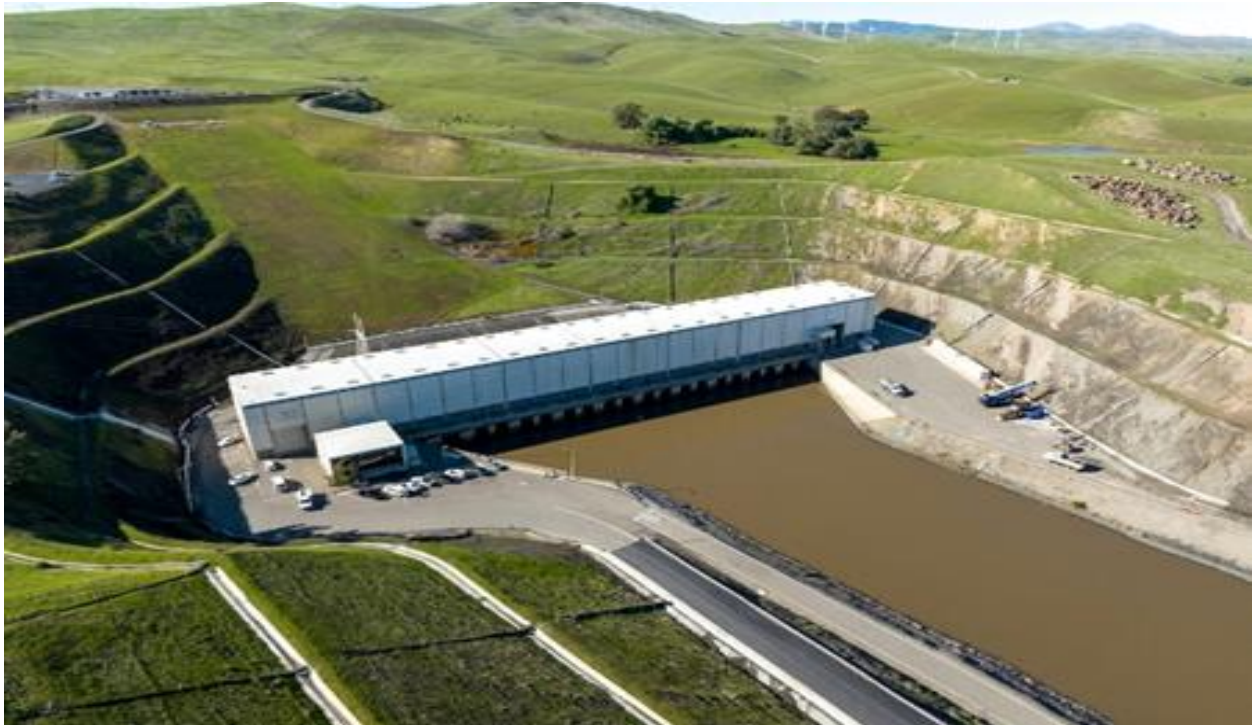
Figure A-39. Picture of Harvey O. Banks Pumping Plant
