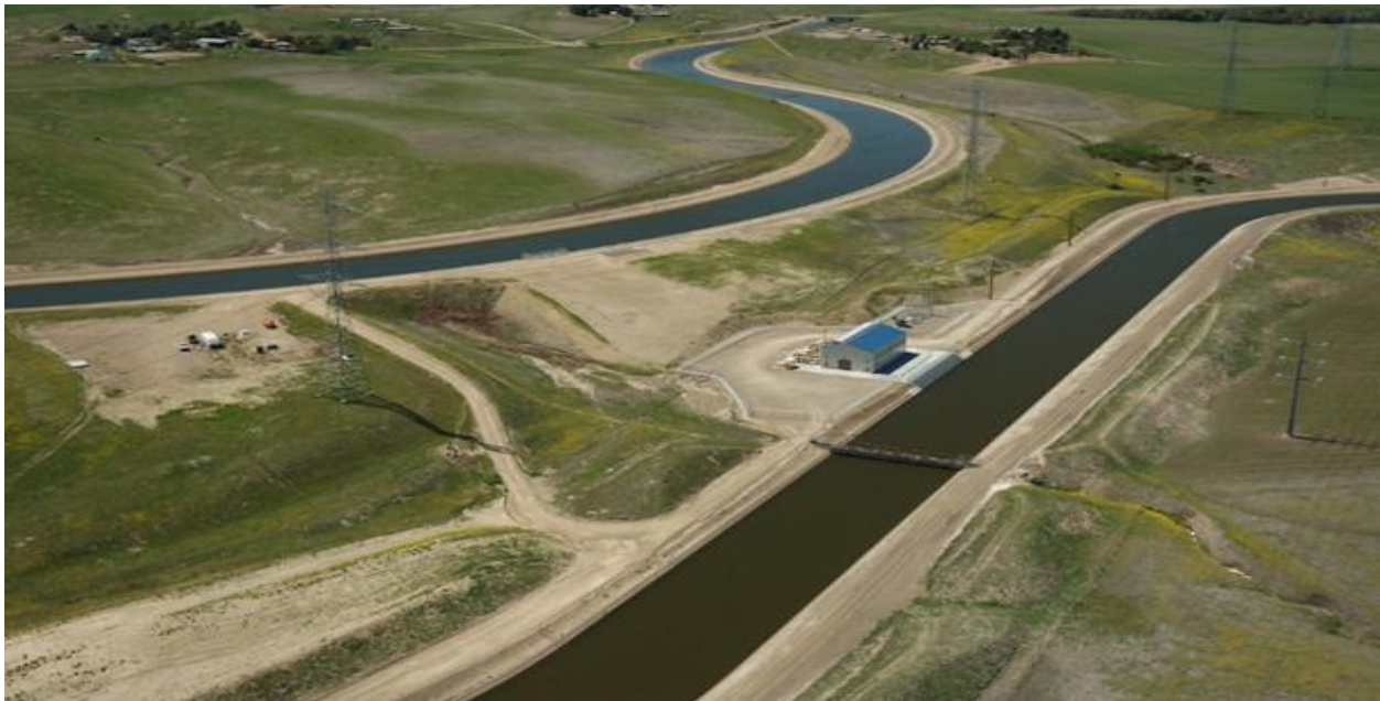
Figure A-15. Picture of Delta-Mendota Canal-California Aqueduct Intertie
