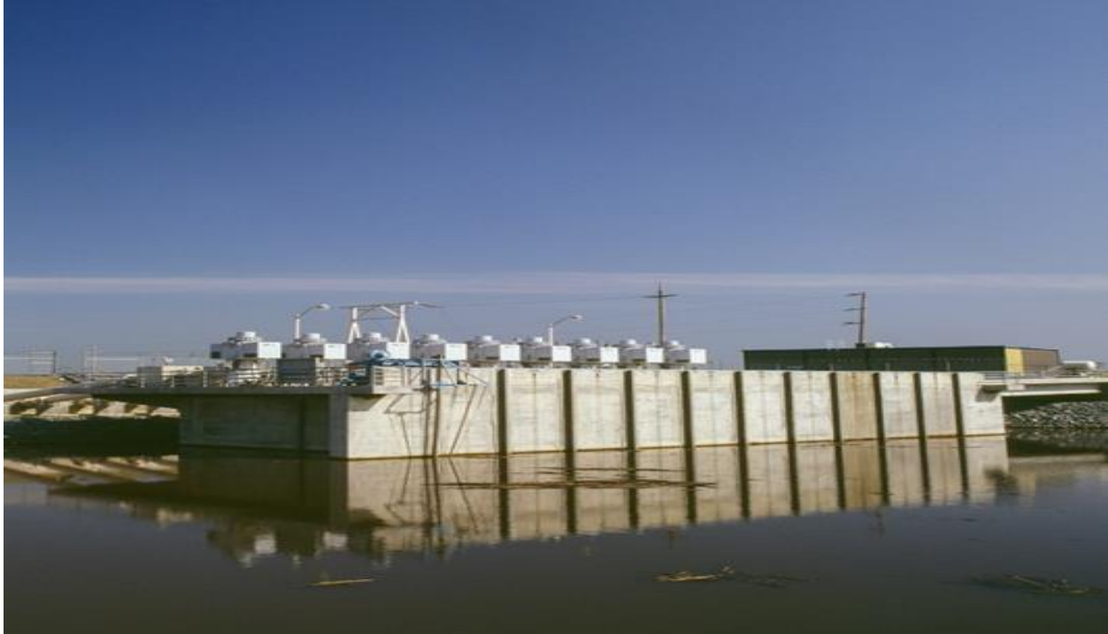
Figure A-41. Picture of Barker Slough Pumping Plant
