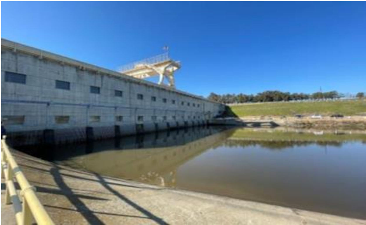
Figure A-11. C.W. "Bill" Jones Pumping Plant
