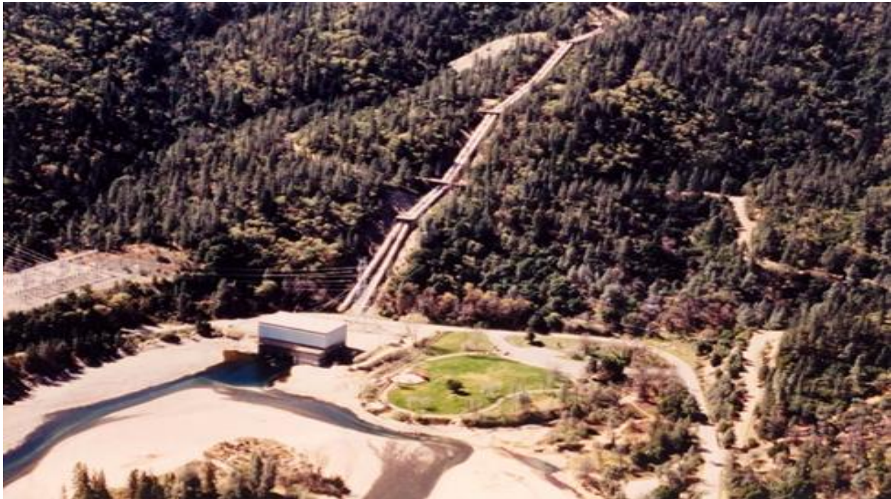
Figure A-32. Picture of Judge Francis Carr Powerhouse
