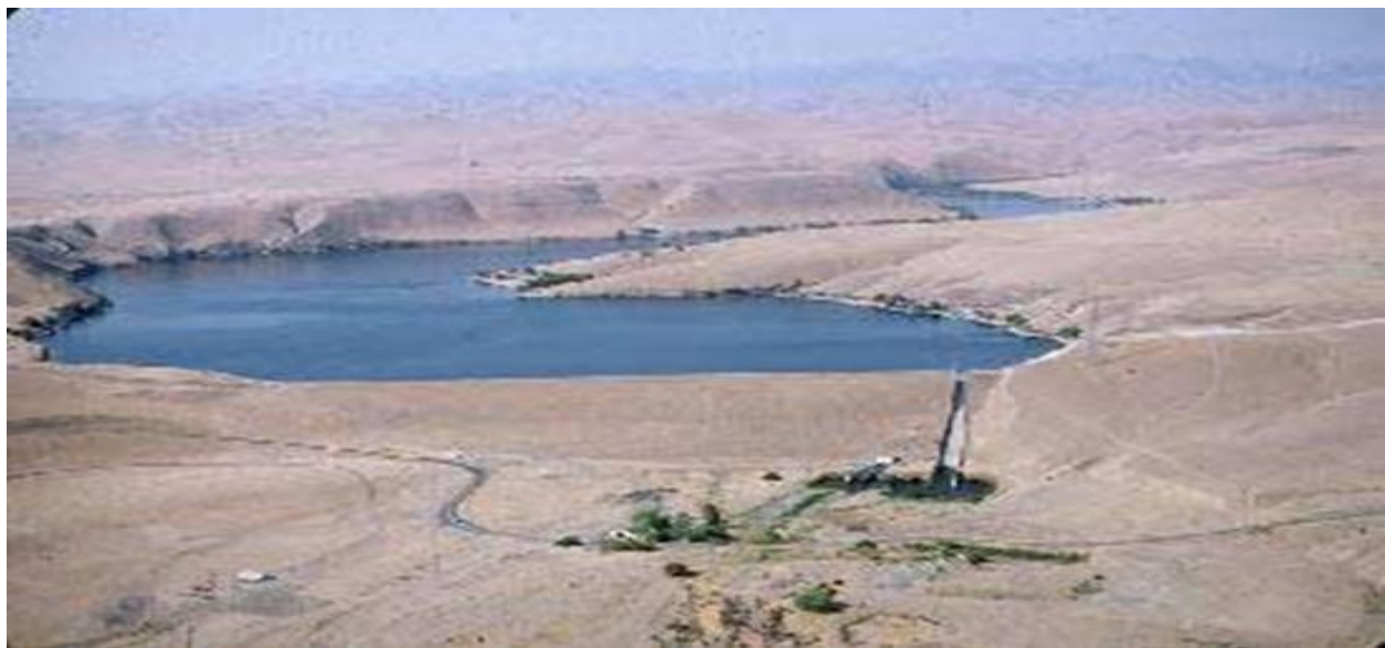
Figure A-37. Picture of Los Banos and Little Panoche Detention Dams and Reservoirs
