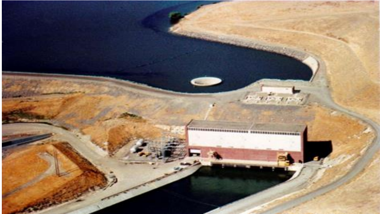
Figure A-35. Picture of O’Neill Pumping Plant
