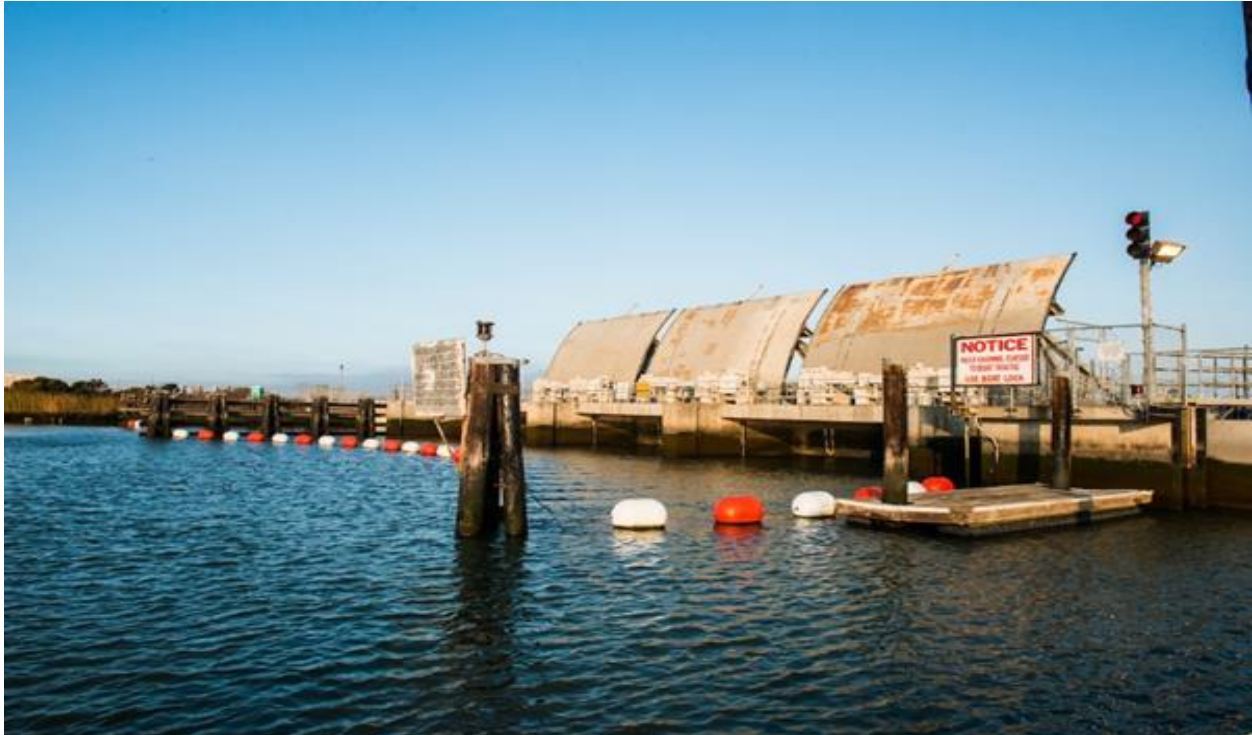
Figure A-42. Picture of Suisun Marsh Salinity Control Gates
