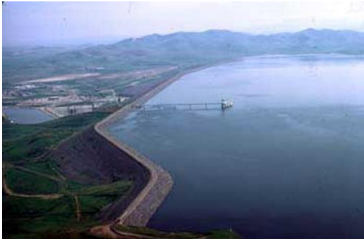
Figure A-34. Picture of B.F. Sisk Dam and San Luis Reservoir
