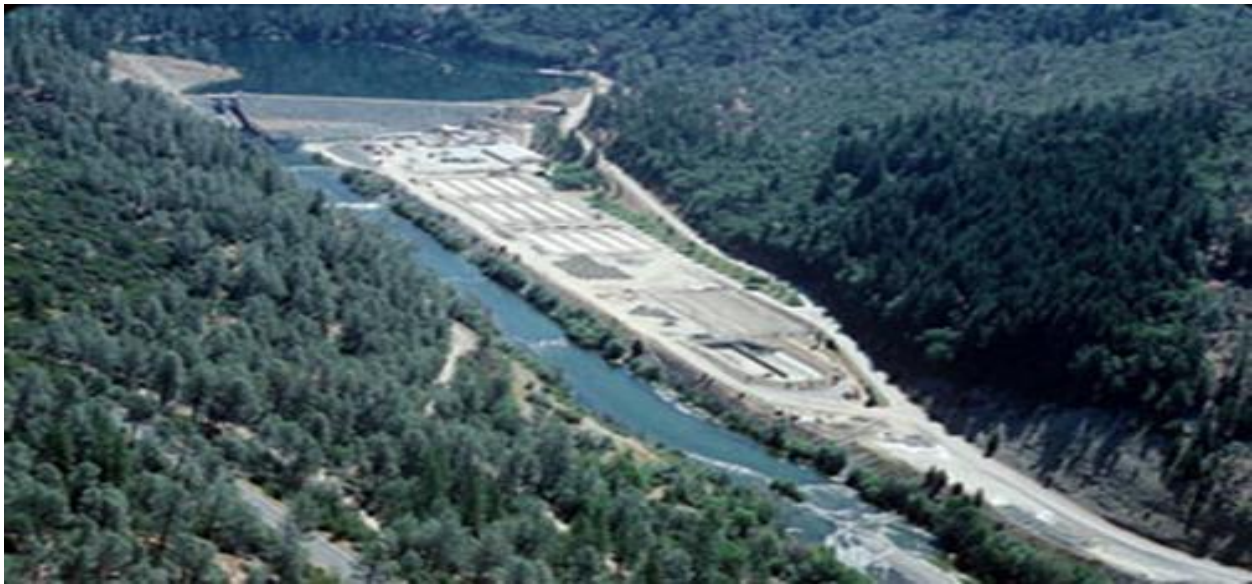
Figure A-31. Picture of Lewiston Dam and Reservoir
