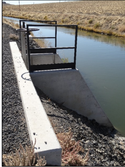
Figure 2. TC-1 turnout structure on the Truckee Canal.
