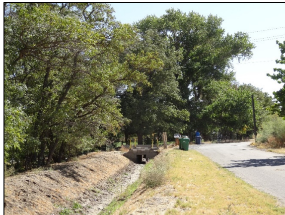
Figure 4. Looking east down the TC-1-1 lateral canal to the box culvert and private road crossing for the proposed pipeline.
