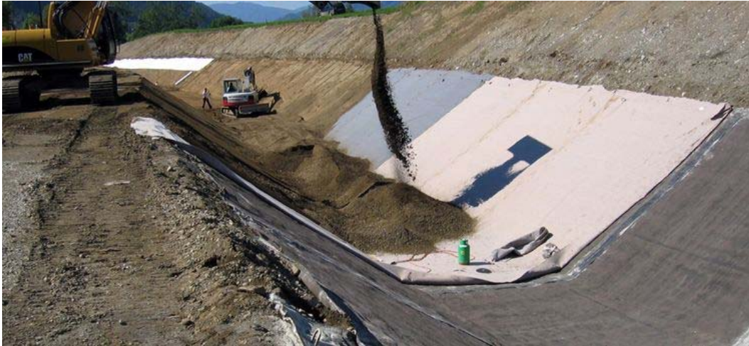
Figure V-6.—Example of geomembrane and soil cover placement. (Huesker, www.huesker.com )
