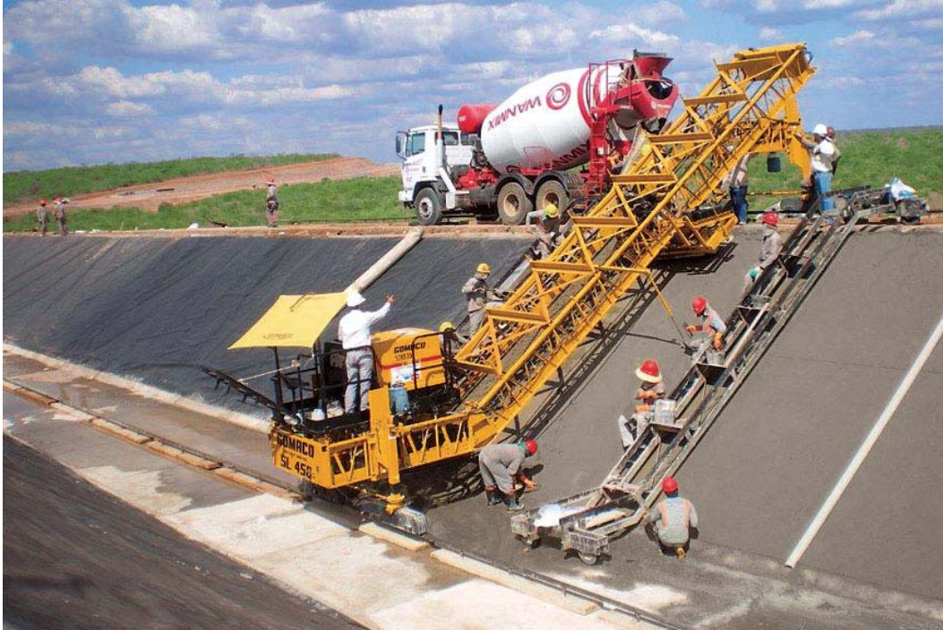
Figure V-4.—Example of partial prism canal paving equipment. (GOMACO, www.gomaco.com )
