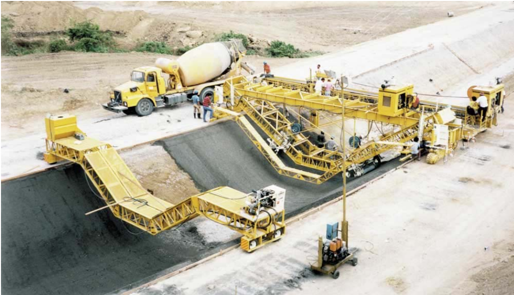
Figure V-2.—Example of full prism canal paving equipment. (GOMACO, www.gomaco.com )
