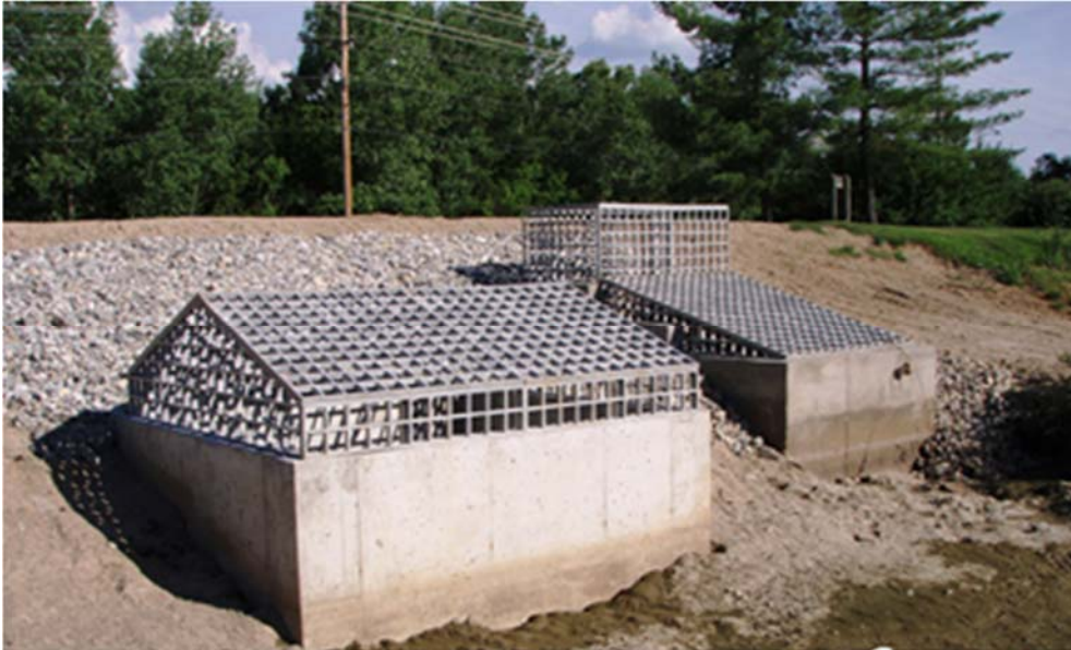
Figure V-19.— Example of trashrack outlet structure.
