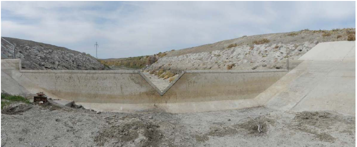
Figure V-24.— Existing Hazen Gauge
