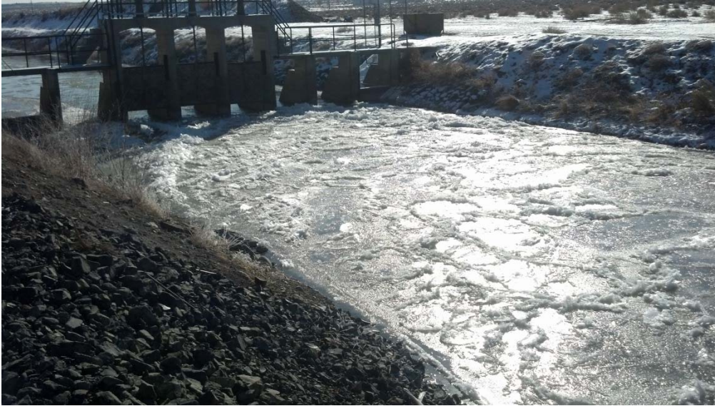
Figure V-11.—Example of ice jams that have occurred historically at the check structure approaches.
