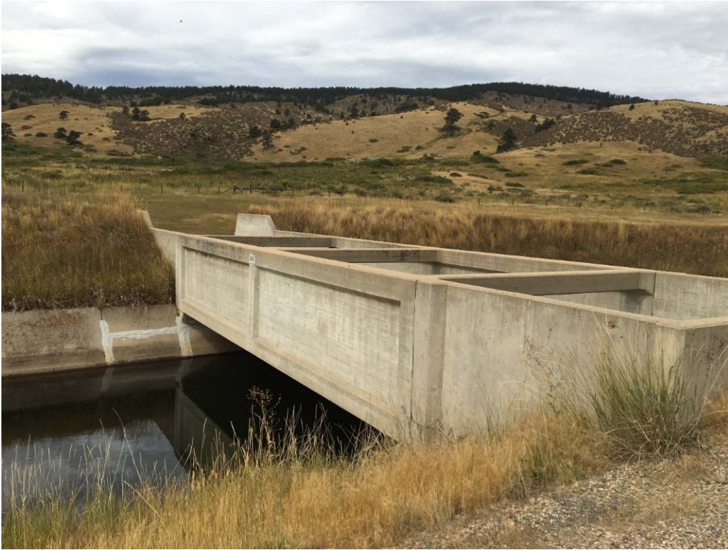
Figure V-14. Example of an Overchute Drainage Crossing.
