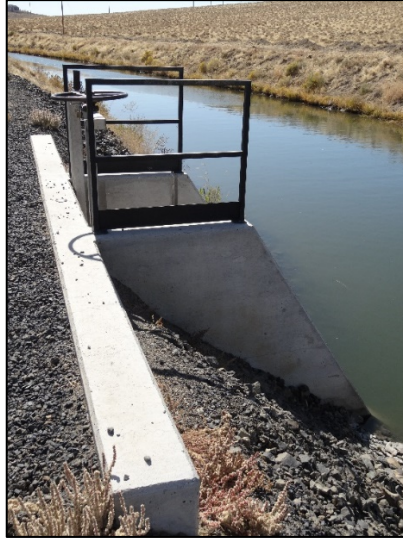
Figure 2. TC-1 turnout structure on the Truckee Canal.
