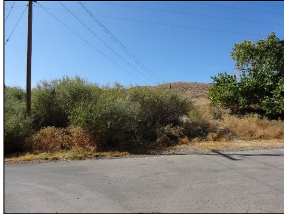
Figure 3. Looking south across Truckee Lane at the proposed sites for the pipeline road crossing and the flowmeter/vault and turnout on the Truckee Canal embankment.
