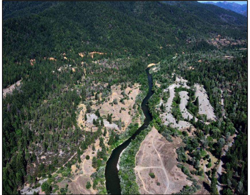
Chapman Ranch Phase A and B project areas before Phase A project construction
