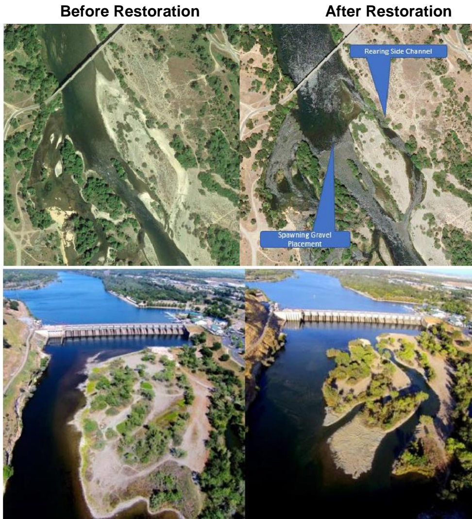
Figure 2-1. Example Floodplain and Side Channel Creation at River Bend (top photos) and Nimbus Basin (bottom photos)
