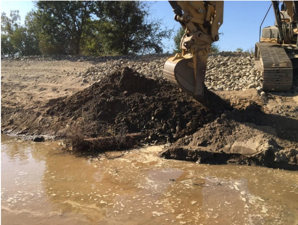
Figure 2-3. Example Woody Material Placement -Sacramento Bar, 2016
