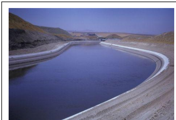
The DMC delivers CVP water from Check 13 located at the San Luis Reservoir to the Mendota Pool. The canal is concrete-lined to its terminus at the Mendota Pool and while it provides fast moving open water habitat, it provides little or no aquatic or emergent vegetation.
