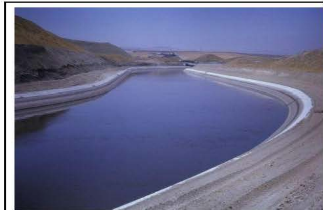
The Delta Mendota Canal (DMC) carries water for 117 miles south to the southern San Joaquin Valley from the Sacramento River Delta and terminates at Mendota Pool. Water would be diverted from the DMC at check 13, more than 40 miles upstream of Mendota Pool, to the O’Neil Forebay of the San Luis Reservoir for delivery to the San Luis Canal and use downstream on MPG farmlands in the San Luis and Westlands Water Districts.
