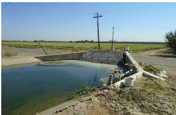
Photo 8. View of the southern terminus of the Weyand Canal, facing east-northeast
