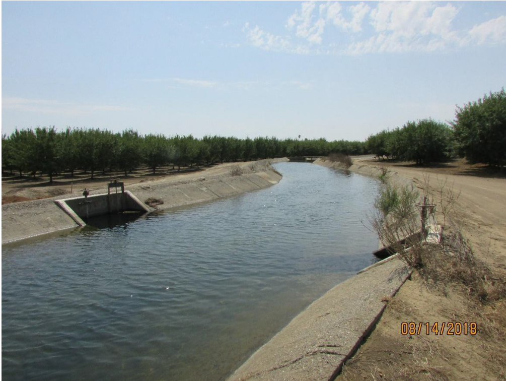
Representative Photograph 6. Lateral/Turnout #6, and Check Structure #4.
