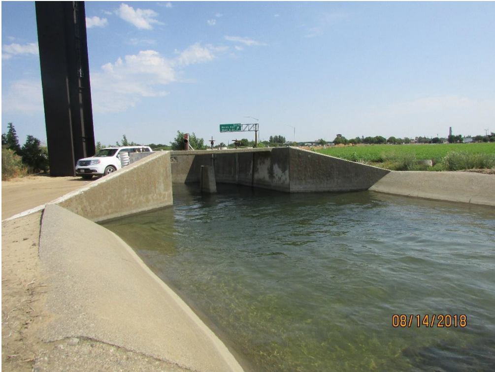
Representative Photograph 3. Lateral/Turnout #2 and #3, and Check Structure #1
