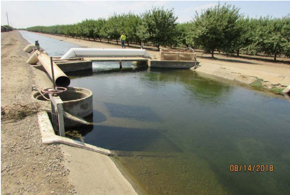
Representative Photograph 7. Lateral/Turnout #7, and Check Structure #3.
