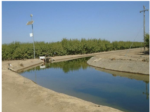
Photo 7. View of the Weyand Canal showing the Lateral 3 headworks and spillway, facing west.
