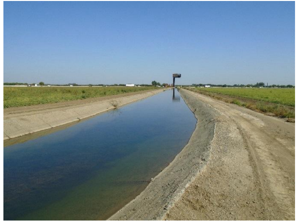
Photo 5. View of the Weyand Canal, facing north.
