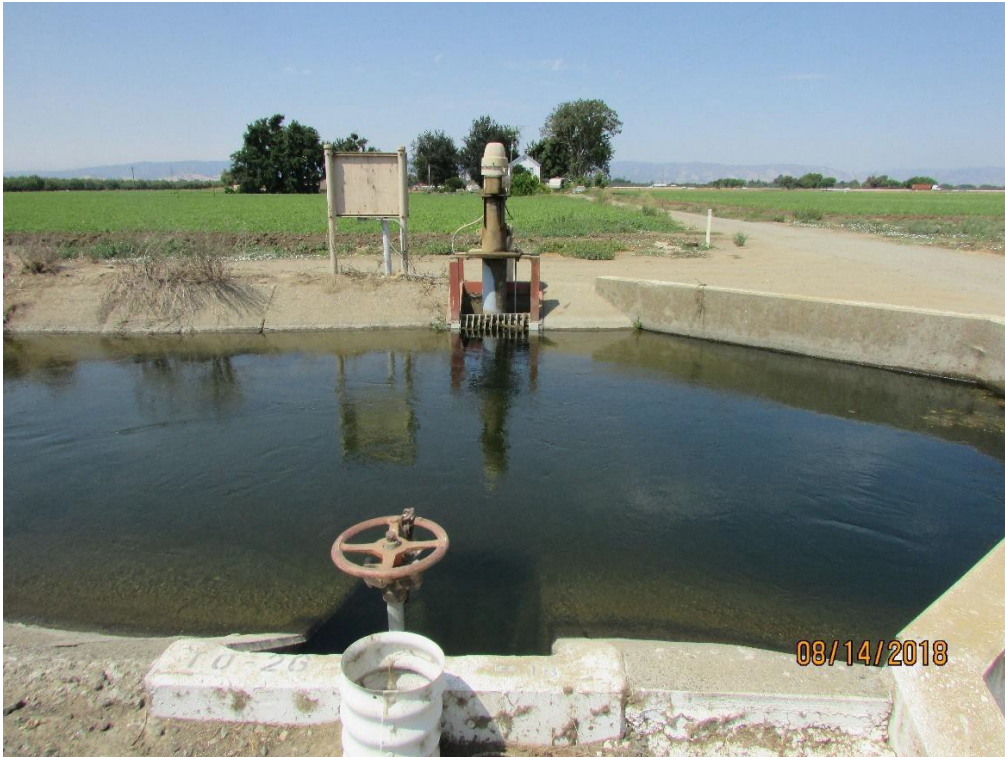
Representative Photograph 5. Lateral/Turnout #5
