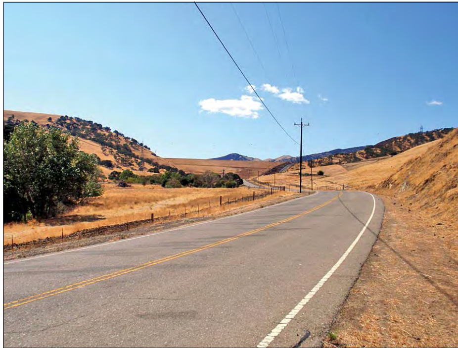
PHOTOGRAPH 1. View from Walnut Boulevard looking southwest at downstream face of the dam. (October 2008)
