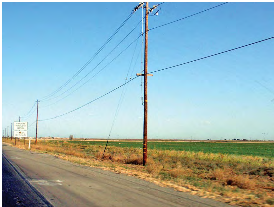
PHOTOGRAPH 8. View from Highway 4 looking southeast along Delta Transfer pipeline alignment (October 2008)
