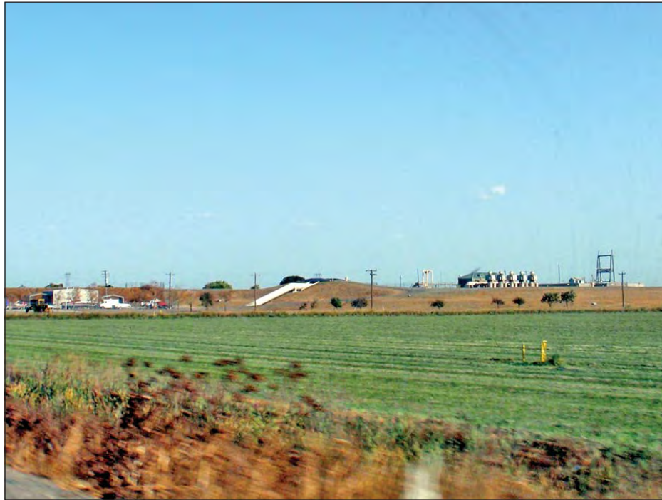
PHOTOGRAPH 7. View from Highway 4 looking east toward Old River Intake and Pump Station (October 2008)
