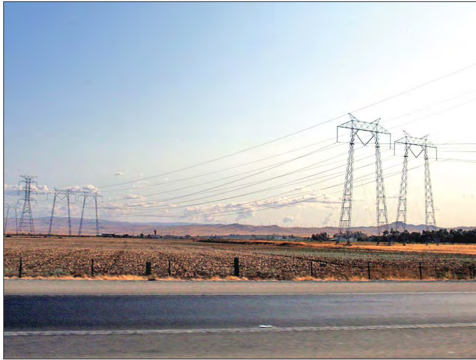
PHOTOGRAPH 9. View from Highway 4 looking southwest along Delta Transfer pipeline alignment (October 2008)
