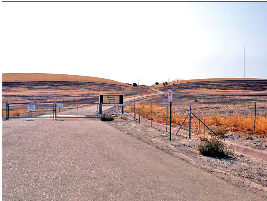
PHOTOGRAPH 10. View from Vasco Road looking southwest along Delta Transfer pipeline alignment to Transfer Facility (October 2008)
