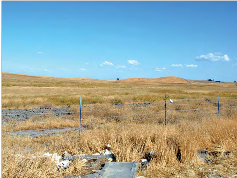
PHOTOGRAPH 13. View from Vasco Road looking southeast toward Transfer-Bethany pipeline alignment (October 2008)
