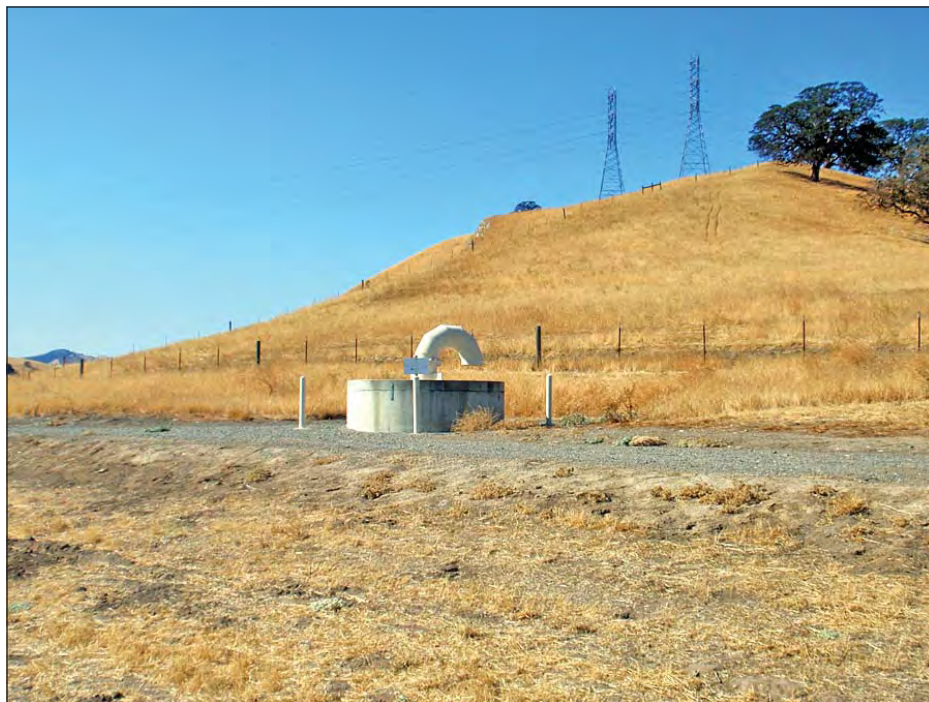
PHOTOGRAPH 14. View from Walnut Boulevard looking west at valve structure of Los Vaqueros pipeline (October 2008)
