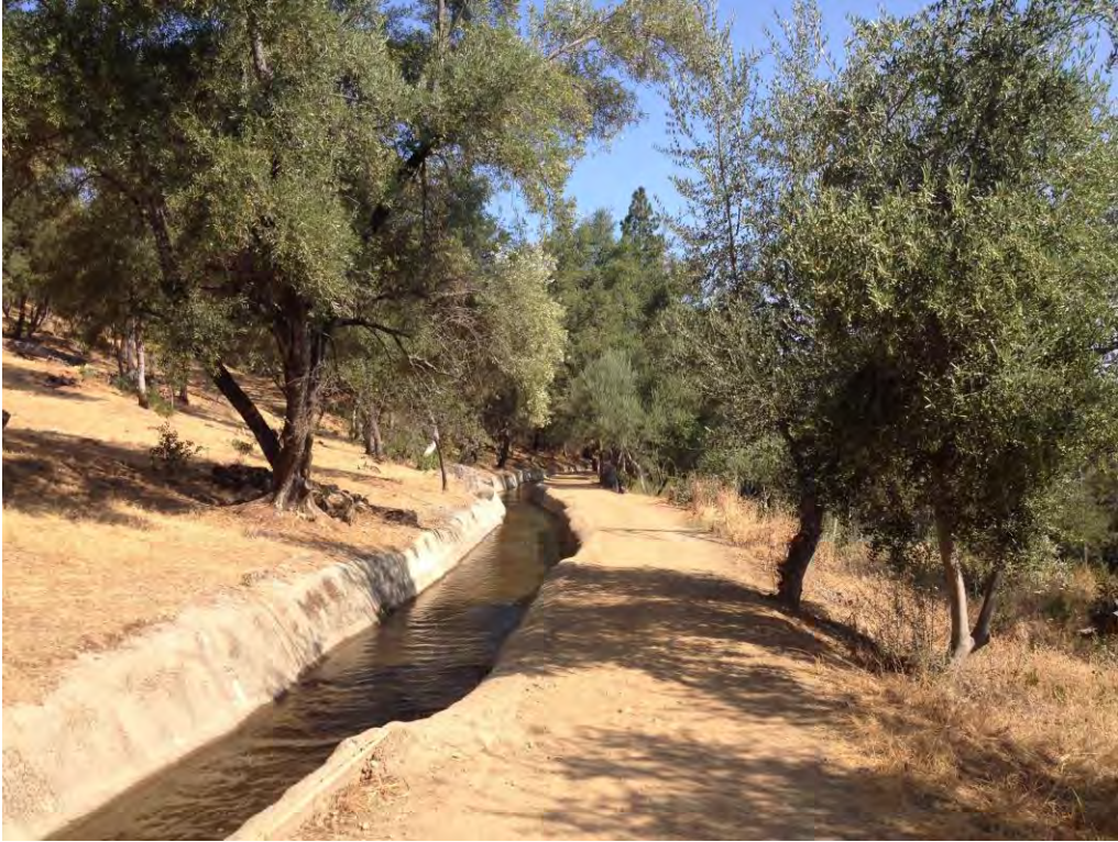
Photo 1 – Shirland Canal through central portion of property
