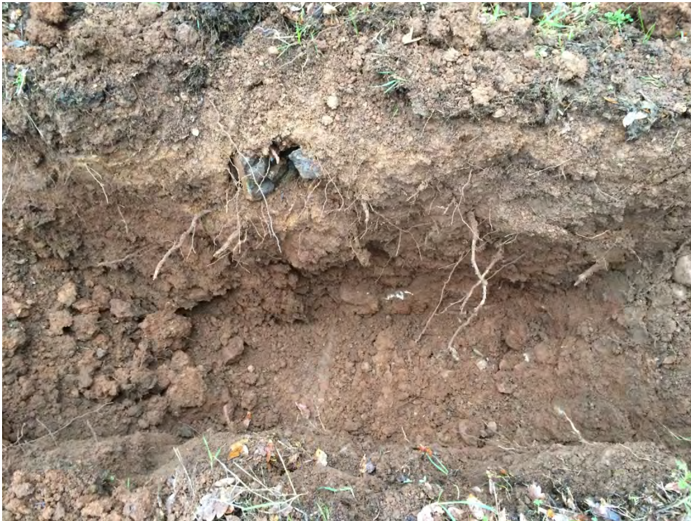
Photo 4 – Fill exposed in exploratory trench T-3.
