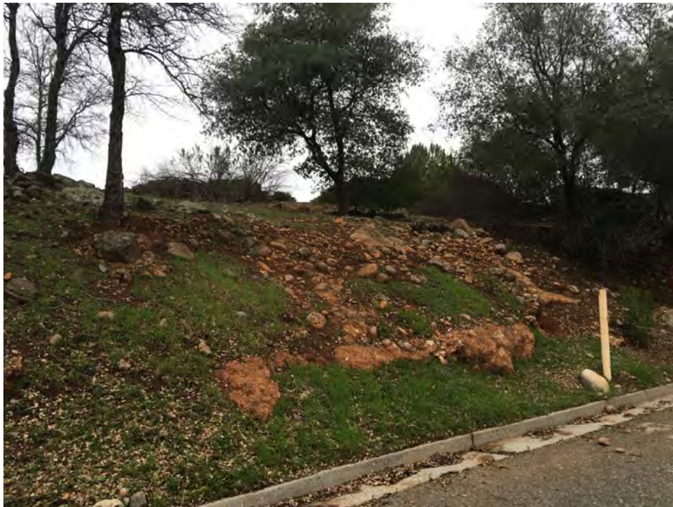
Photo 6 – Mehrten Formation throughout cut slope downgradient of ARD office building.
