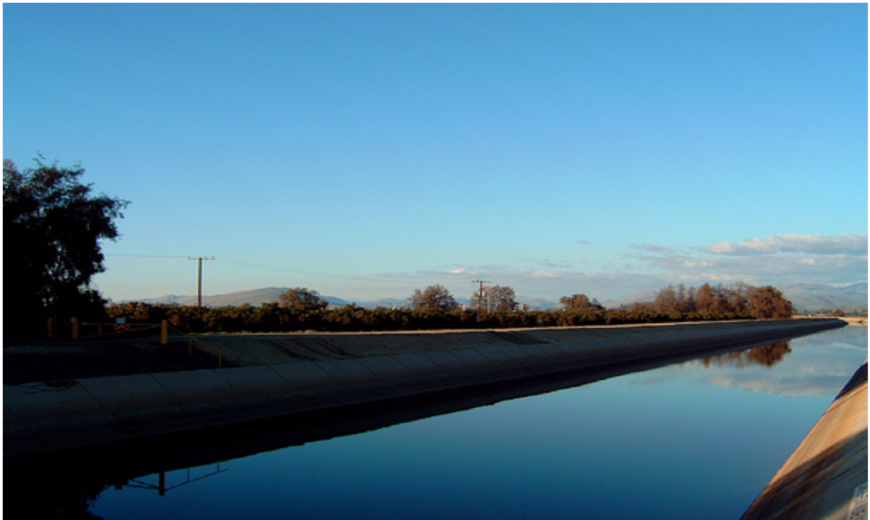
Friant-Kern Canal in Tulare County (Credit: Ted Holzem, Mintier & Associates)
