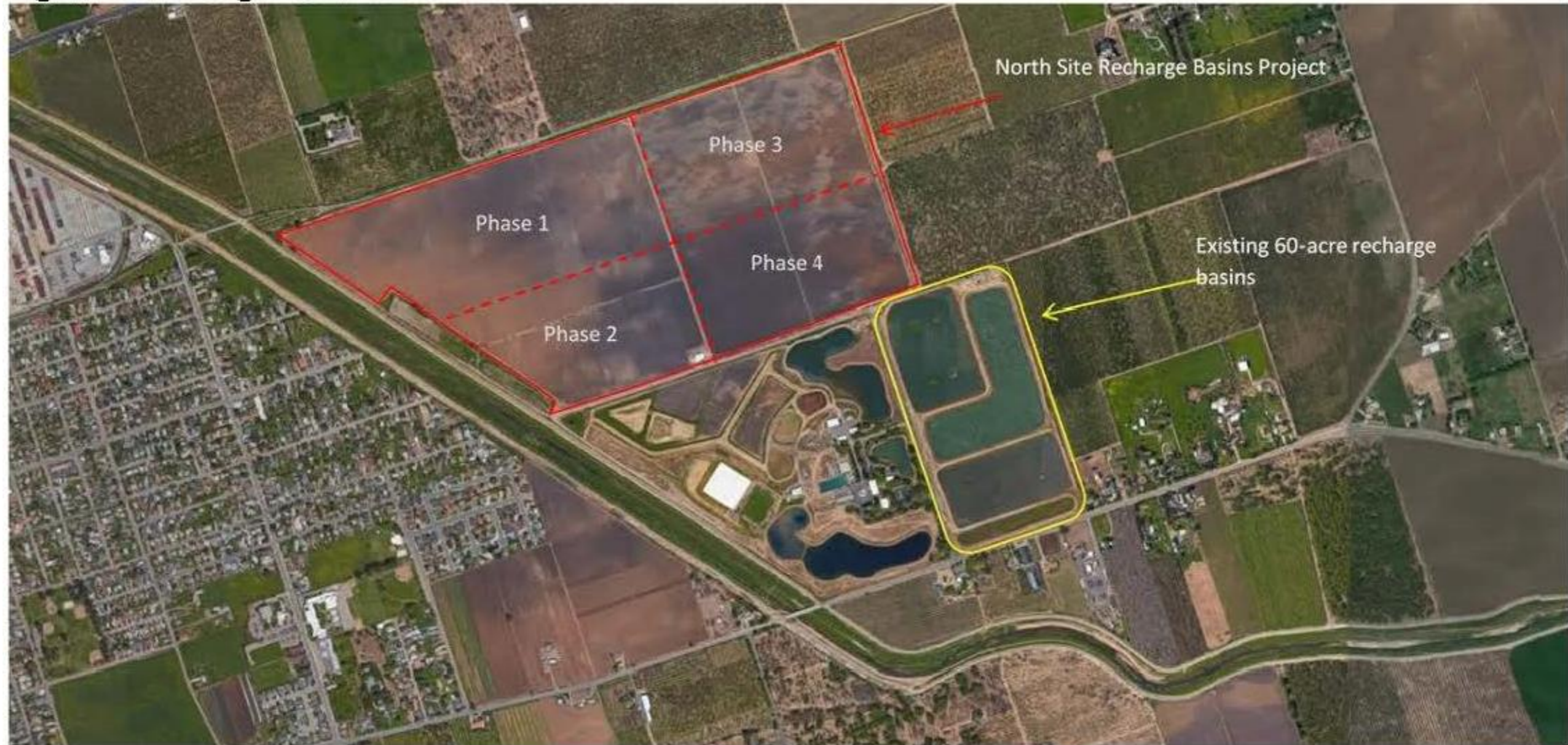
Figure 1. Recharge Basin Site
