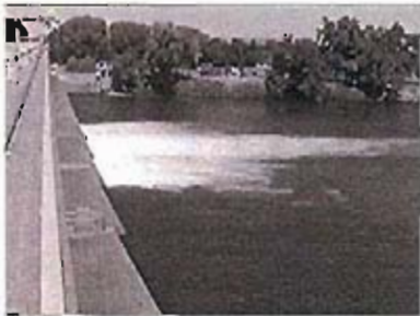
View of white water turbulence downstream of gates 5, 6 and 7. Surface turbulence extended well downstream of the stilling basin endsill.
