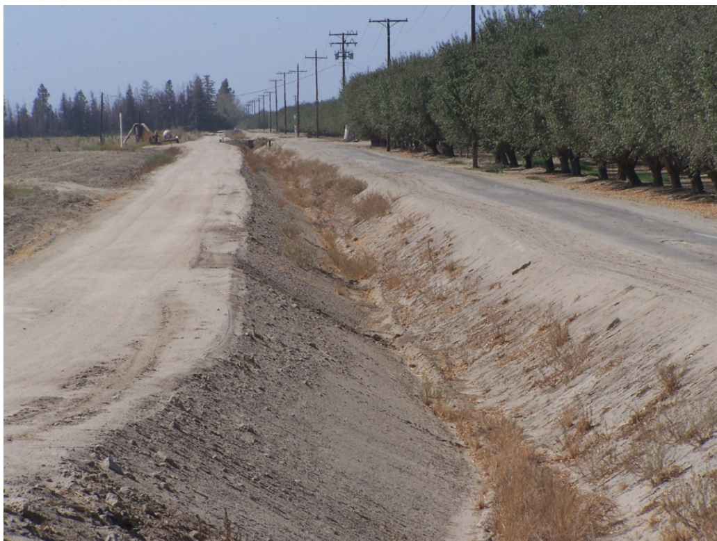
Photograph #8 (below). Earthen-lined Harris Ditch is one of the agricultural ditches of the study area.
