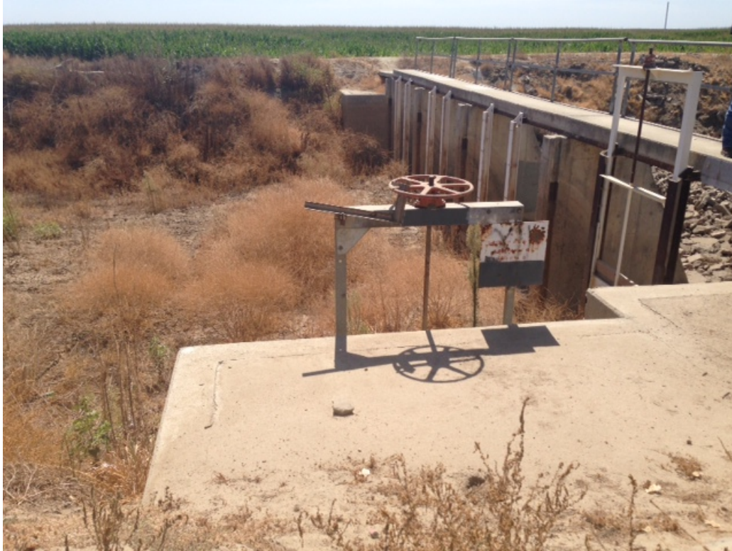
Photograph #7 (above). Another turnout is proposed adjacent to this existing turnout on Deer Creek.
