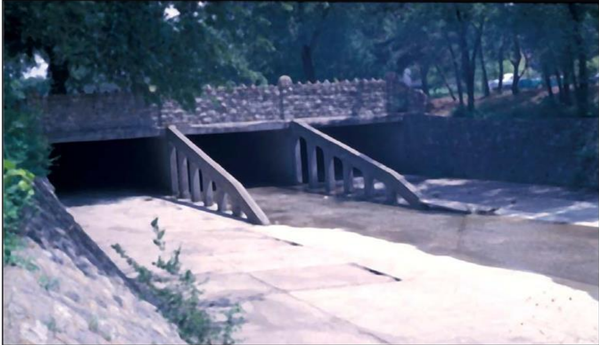
Figure 2-7. Debris Fins Incorporated at Headworks Structure (Example)
