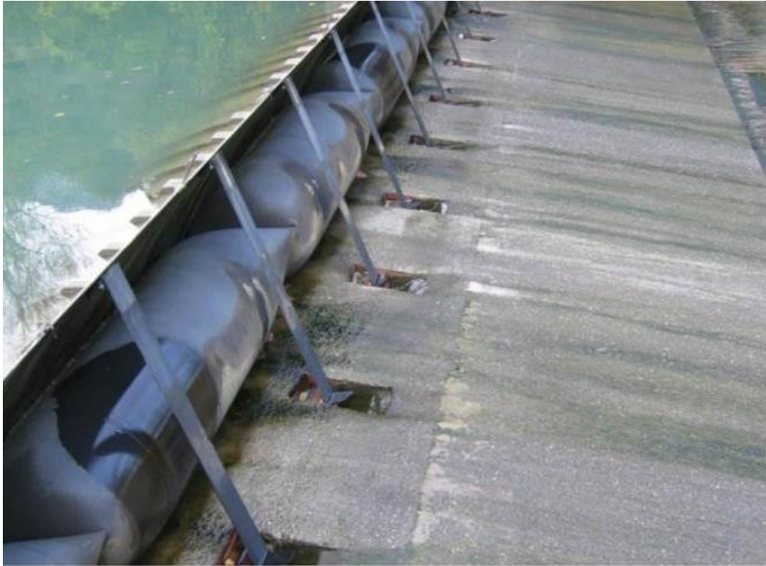
Figure 2-15. Example of Obermeyer-Style Inflatable Gates
