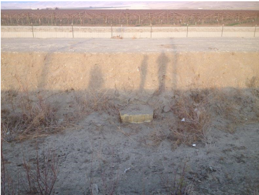
Photo 3 (above): The existing SCA-1 turnout stand pipe and flood channel, which flows adjacent to the South Canal for approximately 1 mile. Photo 4 (below): Reconstruction of the SCA-1 turnout will entail replacing the existing 18” pipe with a 24” pipe; pictured is the approximate location of the existing pipe under the flood channel.
