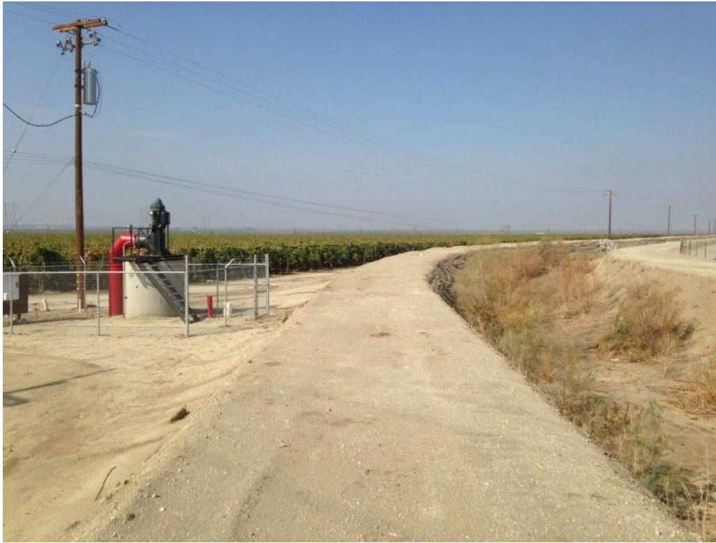
Photo 3 (above): The existing SCA-1 turnout stand pipe and flood channel, which flows adjacent to the South Canal for approximately 1 mile. Photo 4 (below): Reconstruction of the SCA-1 turnout will entail replacing the existing 18” pipe with a 24” pipe; pictured is the approximate location of the existing pipe under the flood channel.
