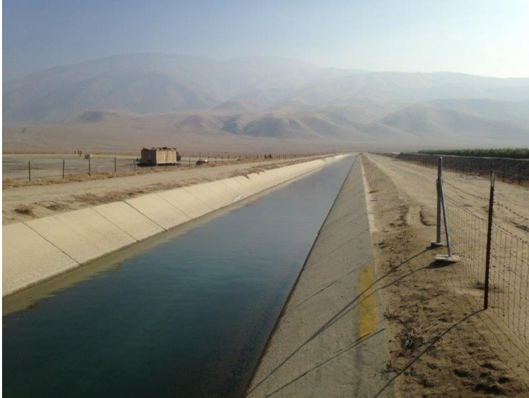
Photo 7 (above): The North and South Canals are engineered, concrete-lined channels; pictured is the South Canal, facing south. Photo 8 (below): The engineered channel of Sycamore Creek that flows through and adjacent to the project site offers limited habitat for native wildlife. Riparian vegetation is absent.
