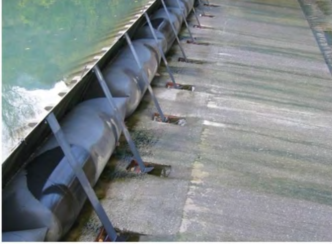
Figure 4-15. Example of Obermeyer-Style Inflatable Gates
