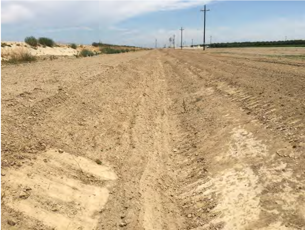
Photo 4: Pond-Poso Spreading and Recovery Facility Conveyance Ditch.
