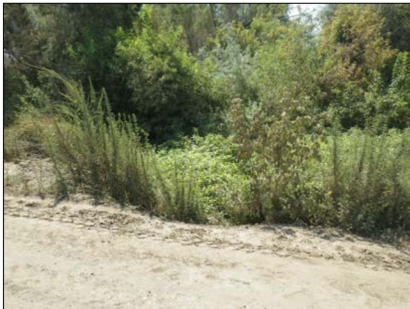
Figure 1-6 View of Downstream Face of Agricultural Road Crossing 2 (Facing South) Showing Vegetation Build-up
