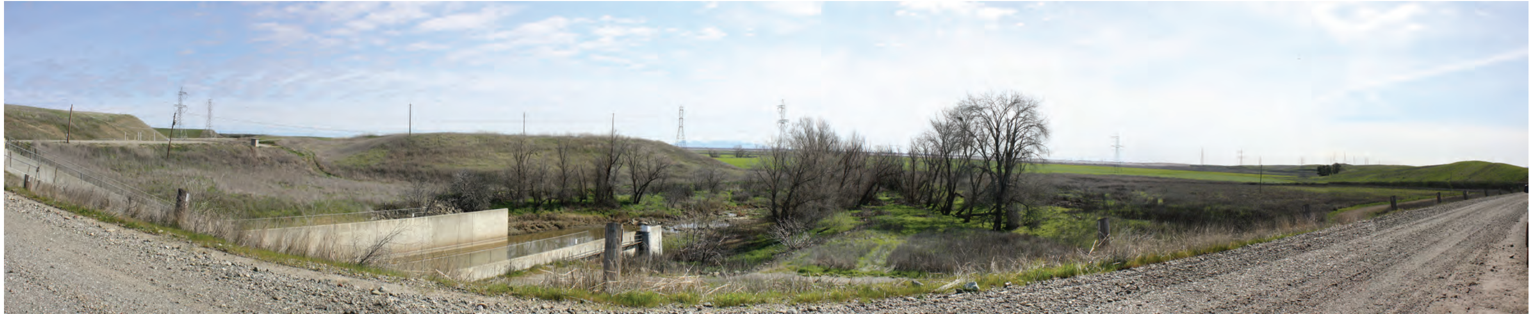
Photo 22: Looking east at the Holthouse Reservoir location from the downstream side of Funks Reservoir near Funks Creek and the Funks Dam Spillway.
