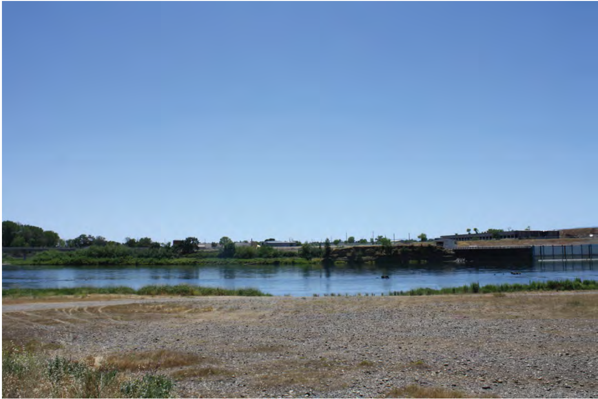
Photo 26: Looking west from the east side of the Sacramento River at the Red Bluff Pumping Plant.
