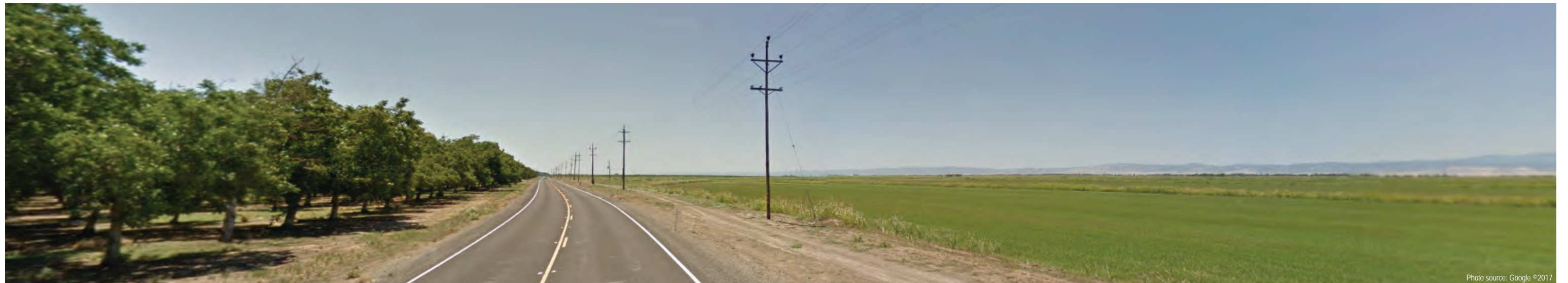
Photo 34: Looking south along the Overhead Power Line (Alternate Alignment), on State Route 45 near Willow Creek Road.
