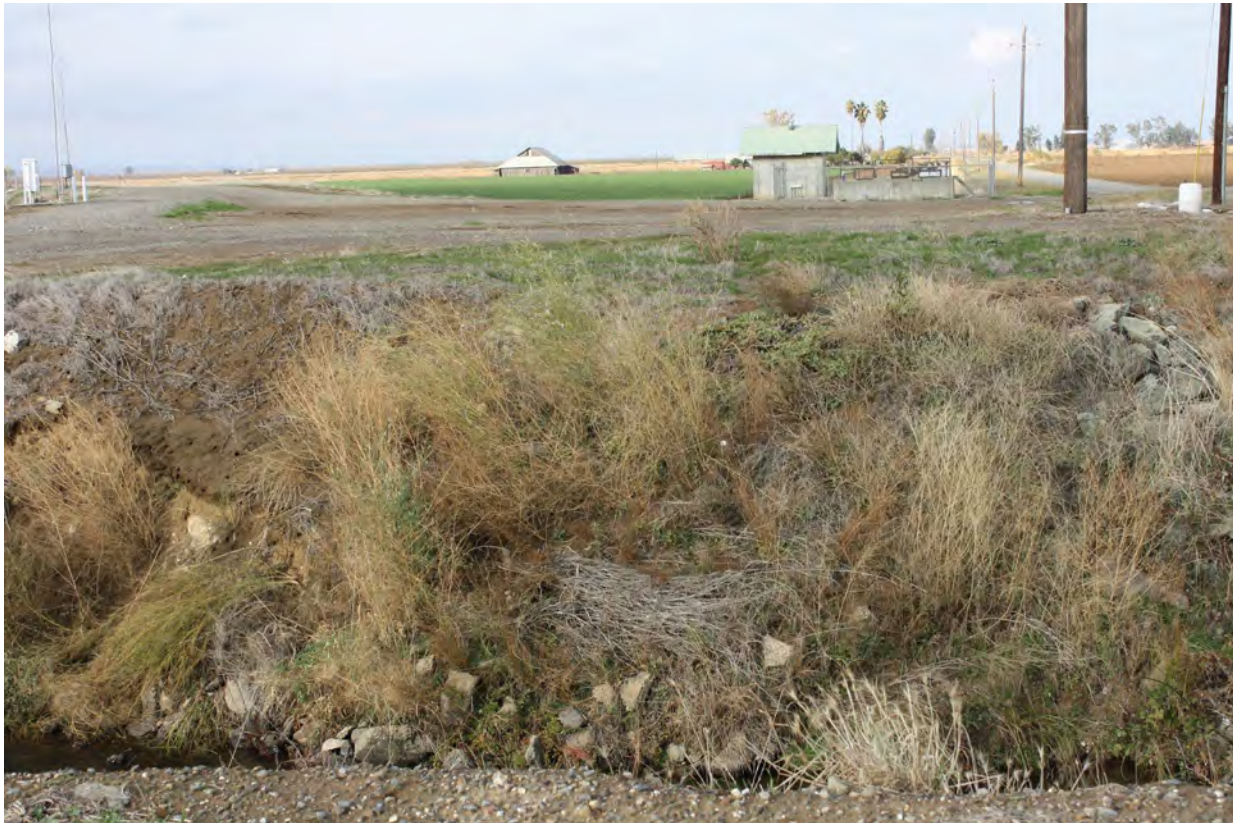
Photo 27: Looking northwest along the alignment of the TRR to Funks Creek Pipeline near the Outlet location at the Funks Creek crossing of McDermott Road.
