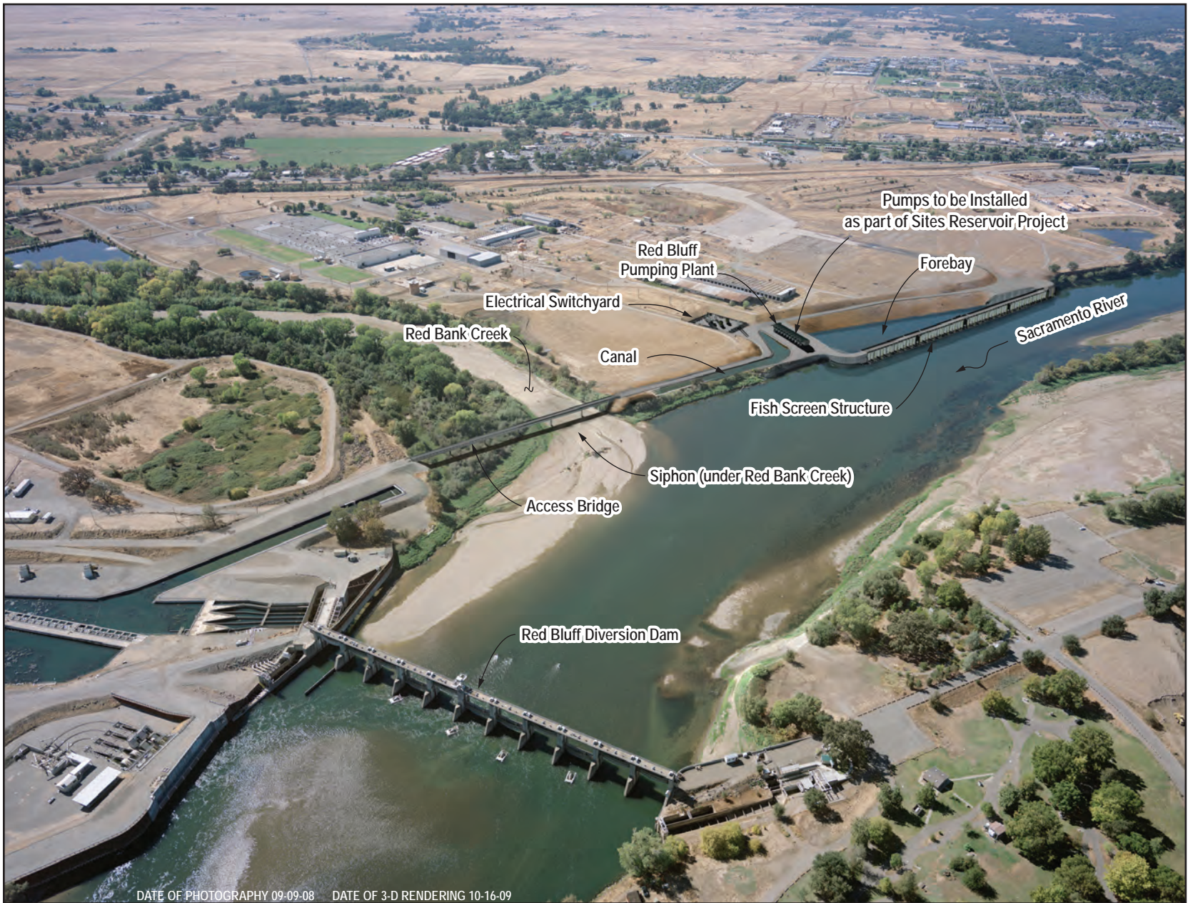
FIGURE 3-11 Location of the Proposed Pump Installation at Red Bluff Pumping Plant Sites Reservoir Project EIR/EIS
