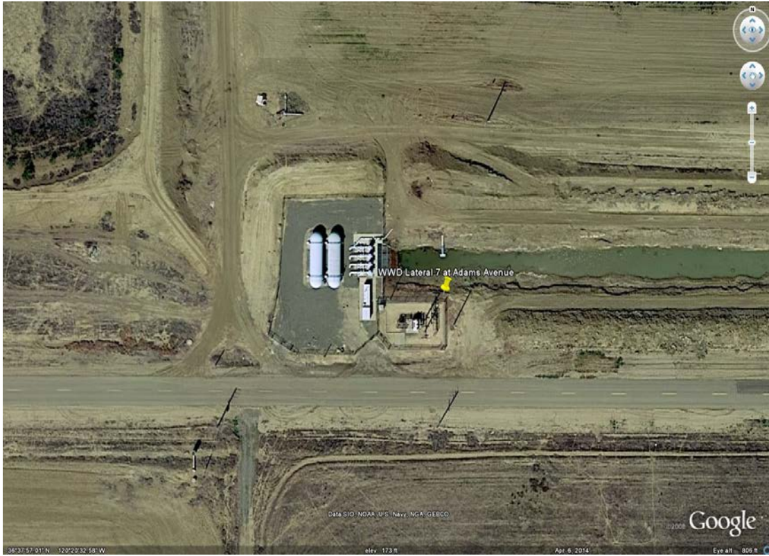
Westlands Water District Lateral 7 at Adams Avenue
