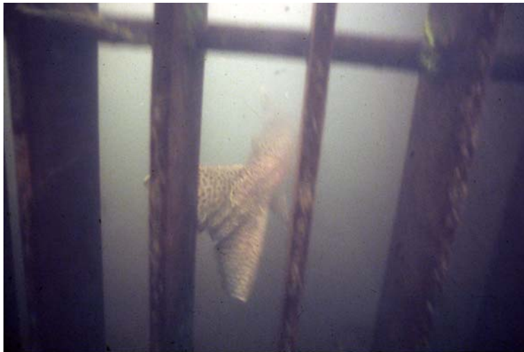
Figure 4. Underwater photograph taken by the author of a chinook salmon trapped inside the bypass terminal box prior to modification of the structure.
