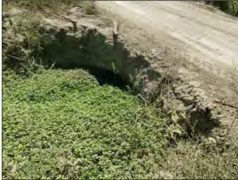
Figure 1-6 View of Downstream Face of Agricultural Road Crossing 2 (Facing South) Showing Vegetation Build-up
