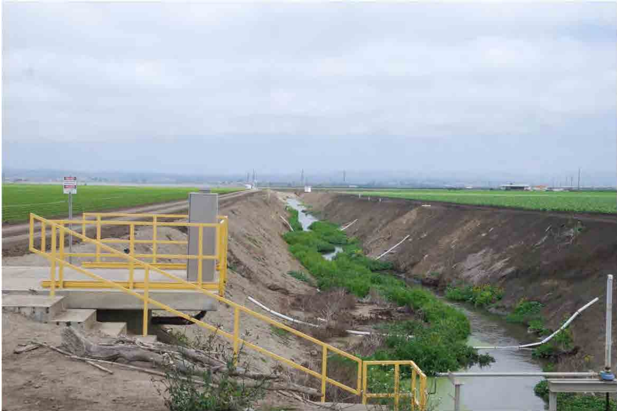
Figure 3-7. Blanco Drain at diversion site looking northeast towards Nashua Road
